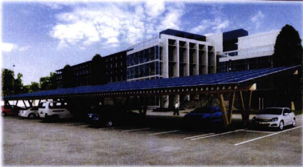
Parking Lot Non-traditional Fix Tilt Solar System
