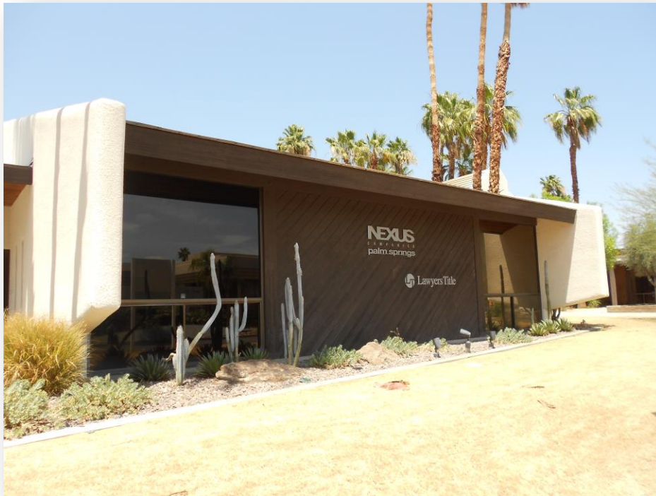
Projecting “fins” provide additional solar protection (Tahquitz Plaza II)
