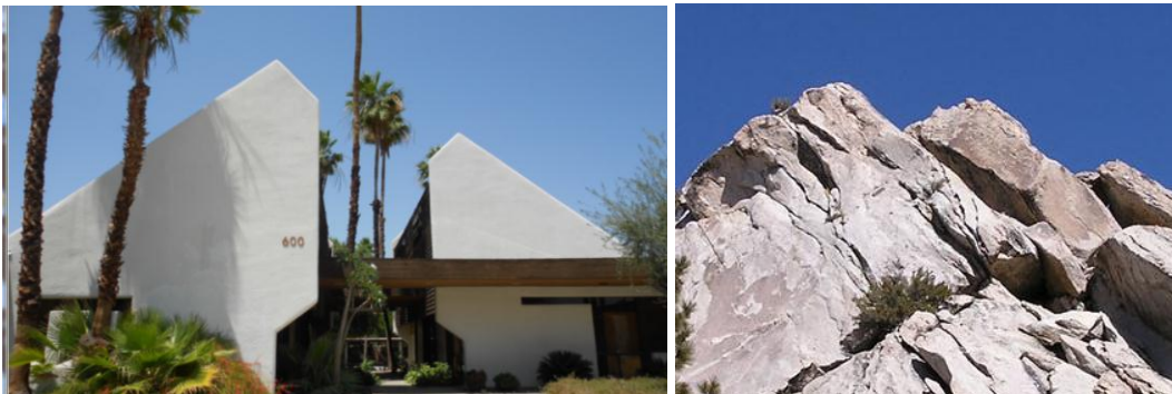
THE STEEPLY PITCHED ROOFS OF TAHQUITZ PLAZA REFLECT THE STEEP SAN JACINTO MOUNTAIN PEAKS NEARBY
