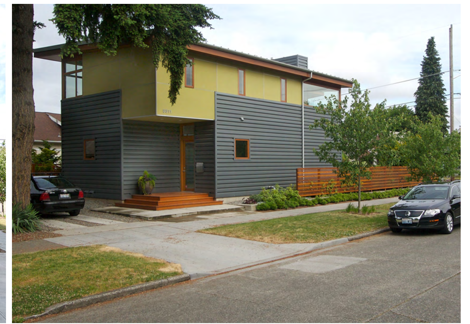
BOXED CORRUGATED GRAY METAL SIDING
