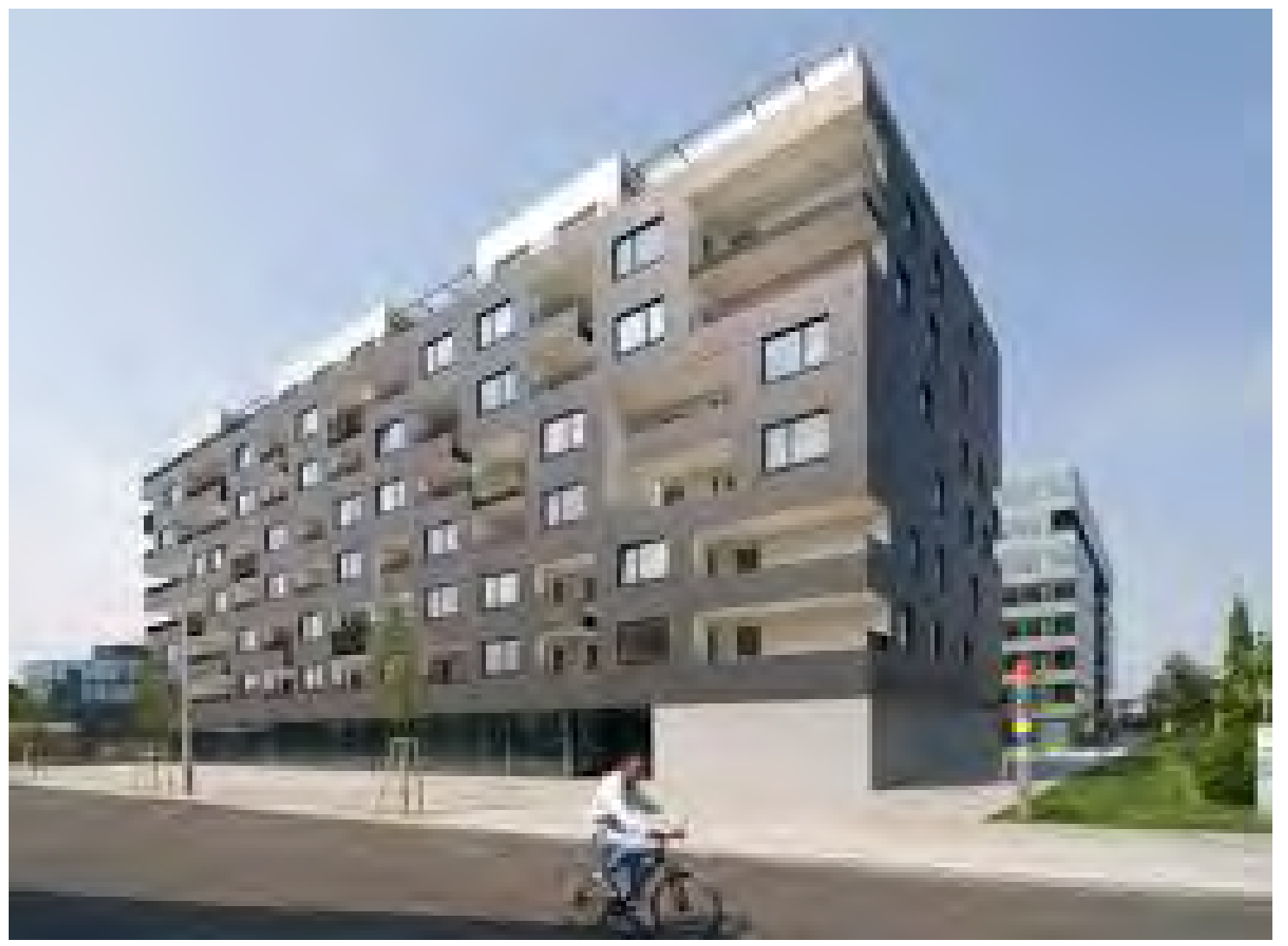
EQUITONE PANEL FACADE
