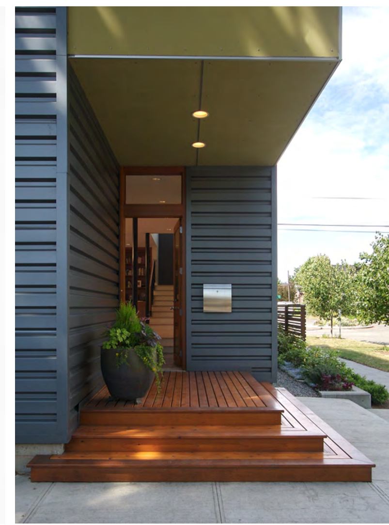
BOXED CORRUGATED GRAY METAL SIDING
