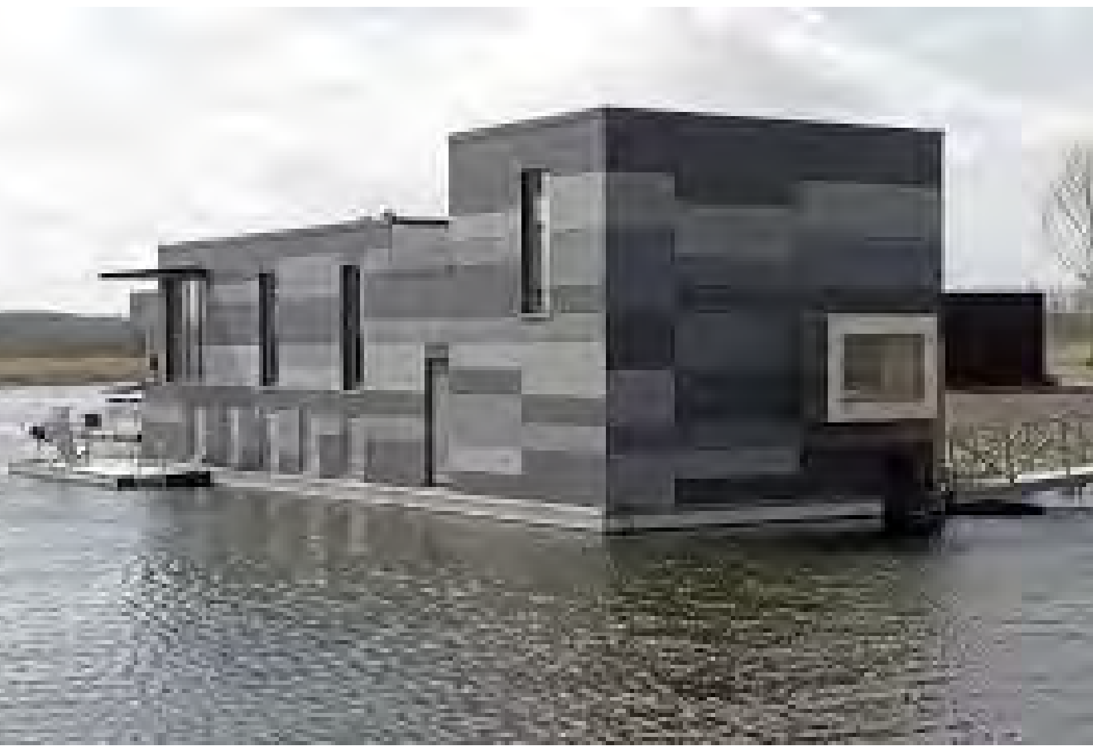
EQUITONE PANEL FACADE
