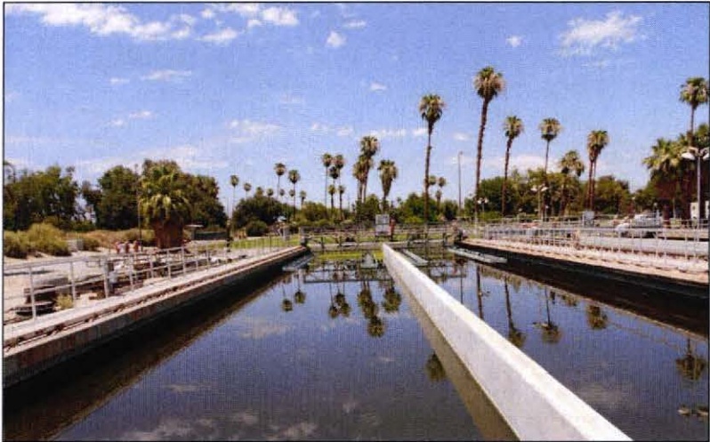
Photo of Palm Trees adjacent to the Secondary Clarifier
