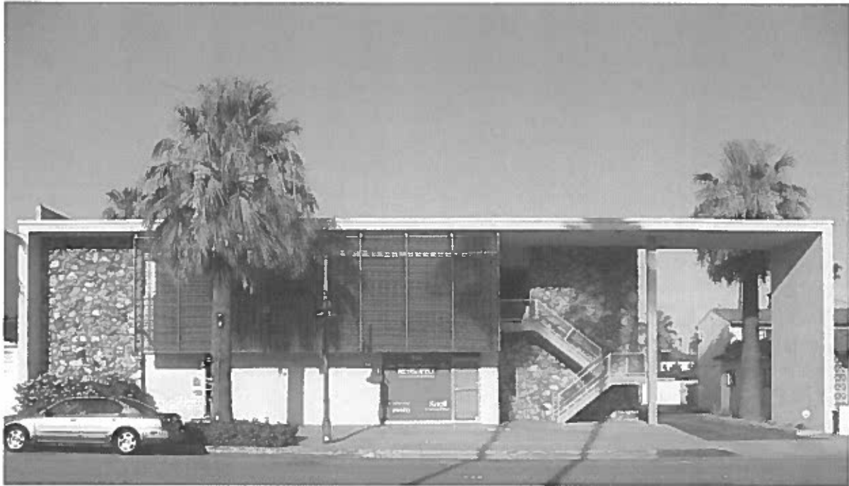
Backstrom-Reid Building (1956, Howard Lapham) 666 North Palm Canyon Drive APN: 50813204
