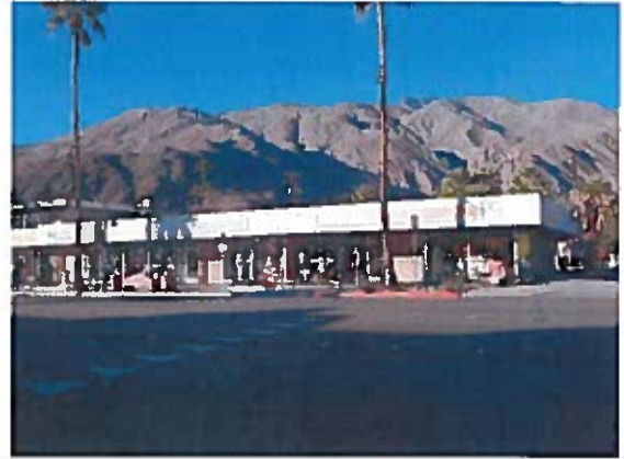
Current Photo Source Historic Resources Group 2014-2015
