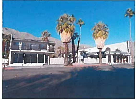
Current Photo Source Historic Resources Group 2014-2015
