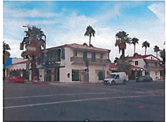
Current Photo Source Historic Resources Group 2014-2015
