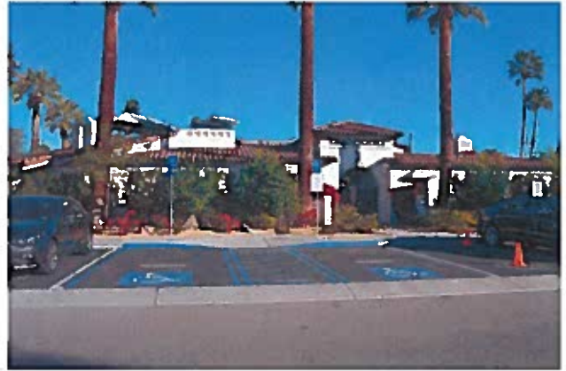
Current Photo Source Historic Resources Group 2014-2015
