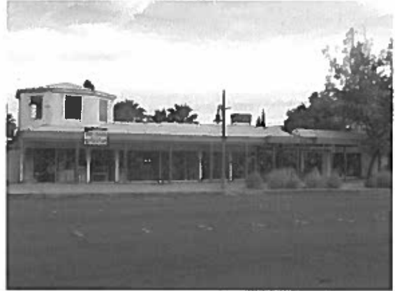
Current Photo Source Historic Resources Group 2014-2015
