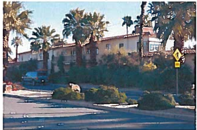
Current Photo Source Historic Resources Group 2014-2015
