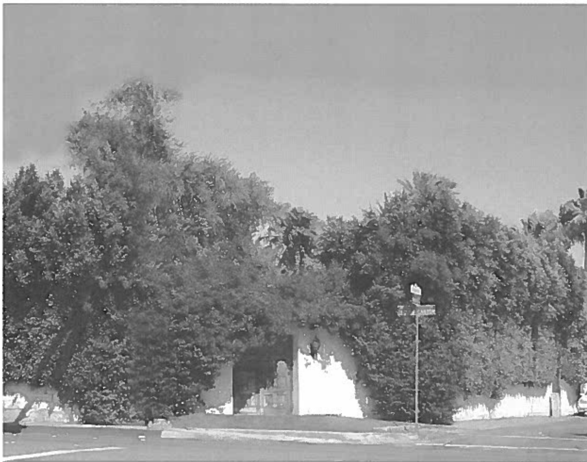
William Schwartz Residence / El Rancho Grande Guest House (1930, Architect Unknown) 814 North Indian Canyon Drive / 200 East Tamarisk Road APN: 567-161-006 Altered
