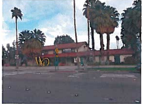
Current Photo Source Historic Resources Group 2014-2015
