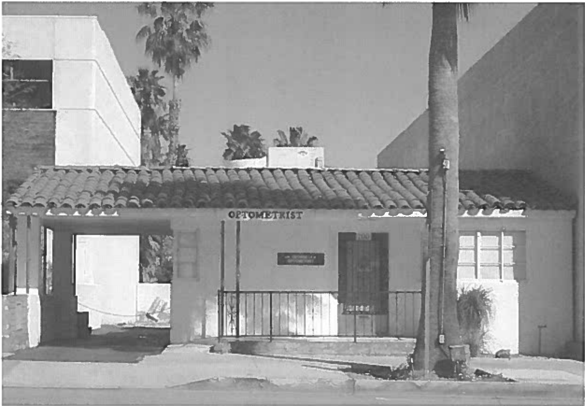
Clifton Dental Building / Purcell Building (c. 1937, John Porter Clark) 700 North Palm Canyon Drive APN: 505-303-002
