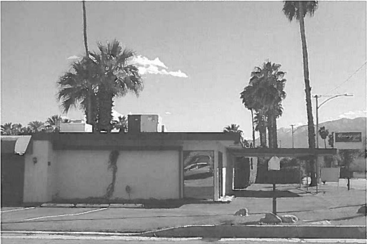
Lubenski Apartments / Morningside Inn / Bear Resort (1943, Architect Unknown) 888 North Indian Canyon APN: 507-161-001
