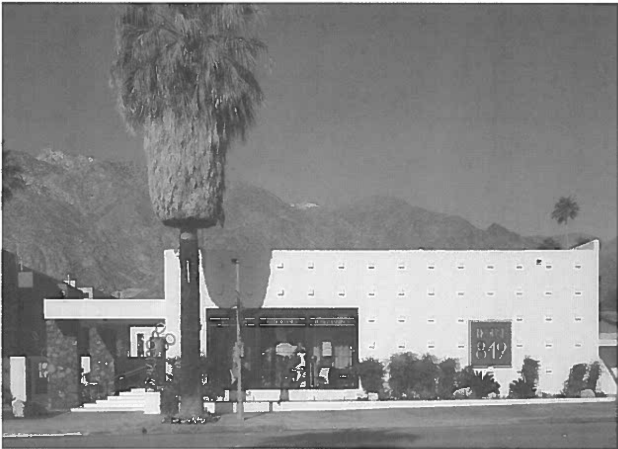
US Post Office / House 849 (1955, Architect Unknown, alts 2005, Dean Carlson) 849 North Palm Canyon Drive APN: 505-283-010
