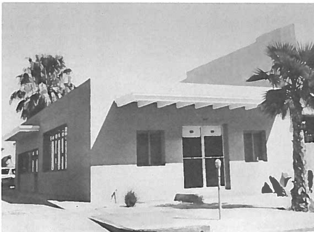
Palm Springs Water Company (1941, John Porter Clark) Altered 844 Palm Canyon Drive. [Contemporary] APN: 505-285-006
