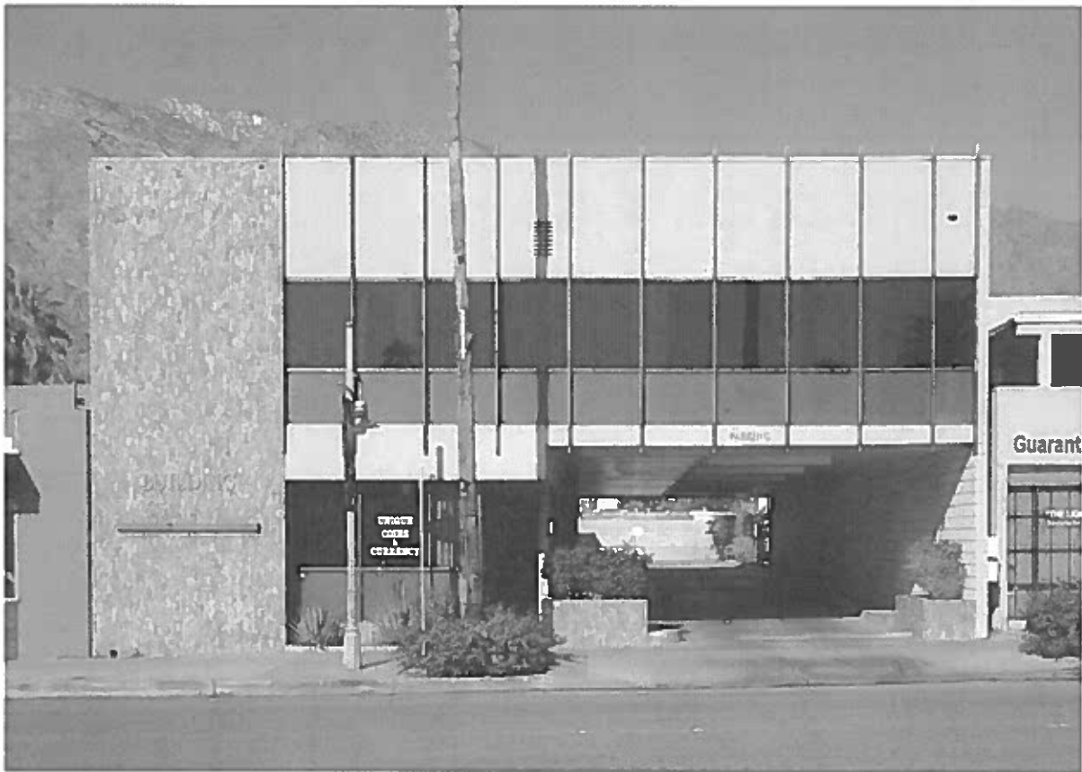
Holloway Building (1970, Stan Sackley) 655 North Palm Canyon Drive APN: 505-302-011
