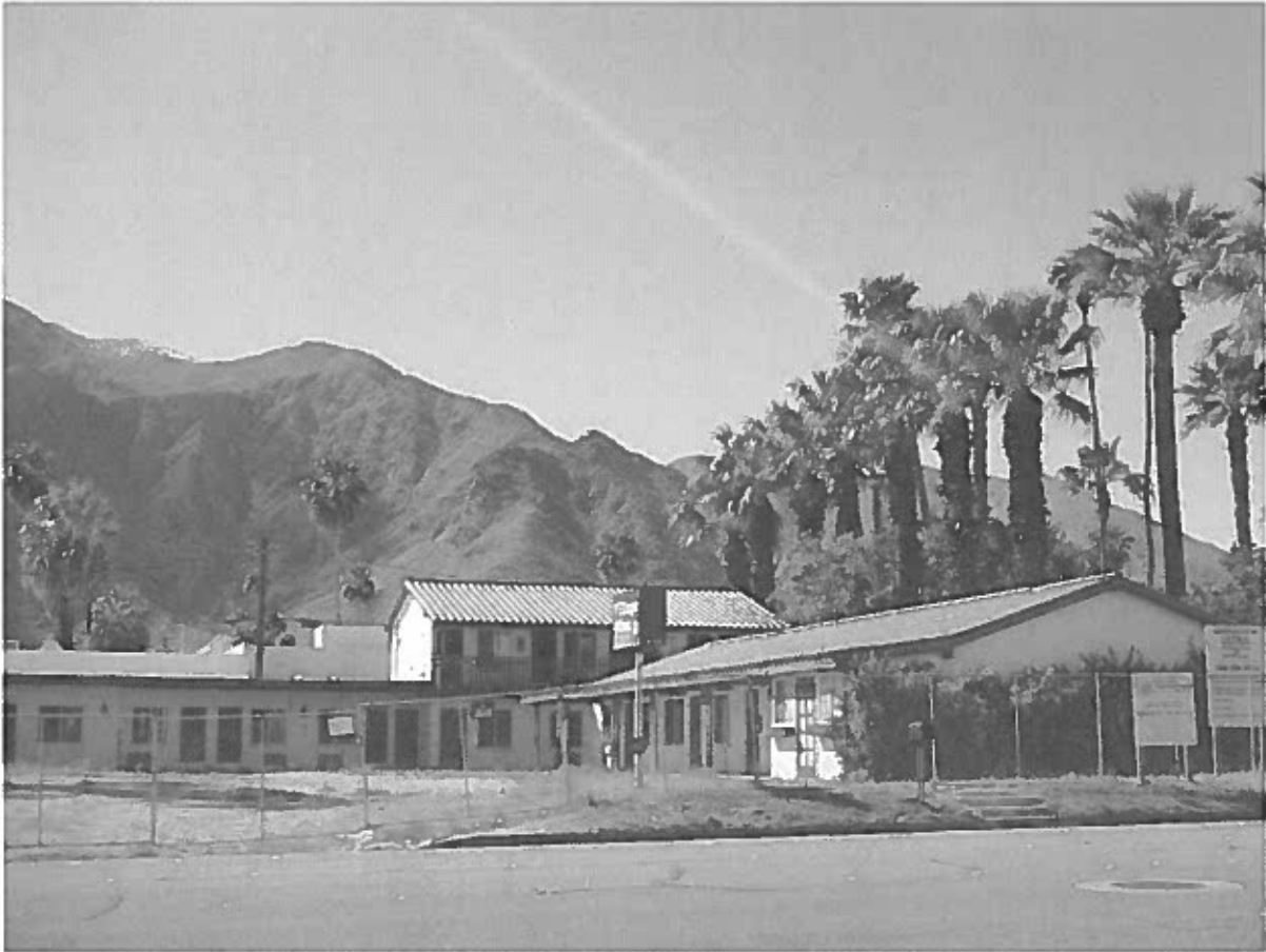
Crawford Apartments / Village Inn (1945, Architect Unknown; Henry Samarian, Builder) 855 North Indian Canyon Drive APN: 505-285-01
