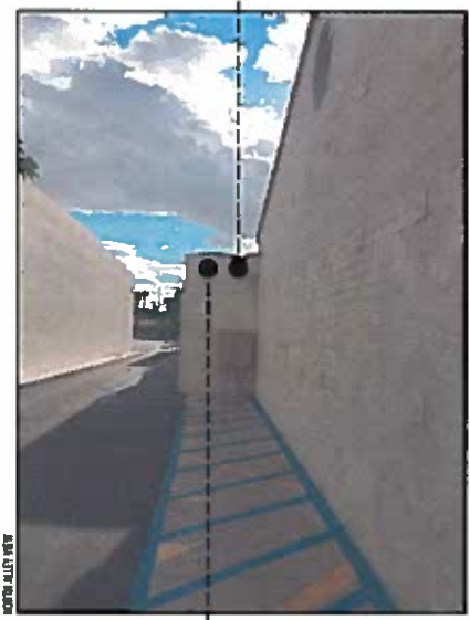
EXISTING MECHANICAL PLATFORM
