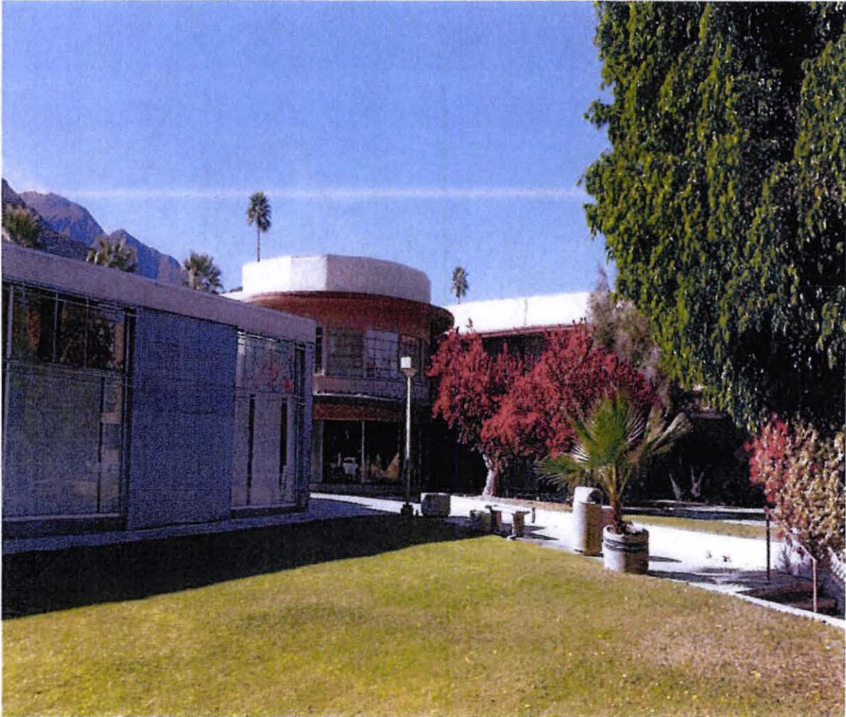
Photo 10. In the courtyard looking northwest toward Building E with Building A in background, March 2015
