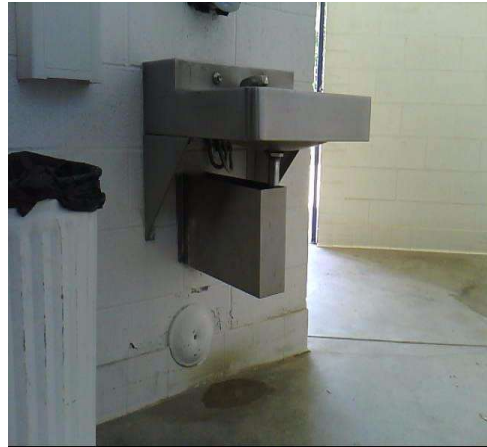
Restroom , Lavatory : Lavatory - Supply Lines not wrapped
