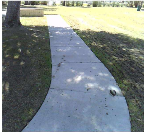
Path Of Travel , Walking Surfaces : Change in Level
