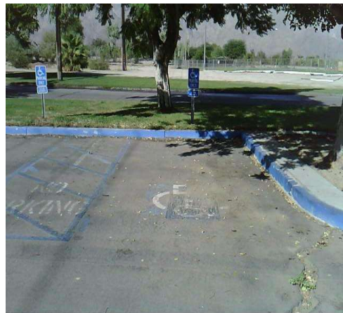
Parking Lot , Parking Space : ISA is Faded or Damaged
