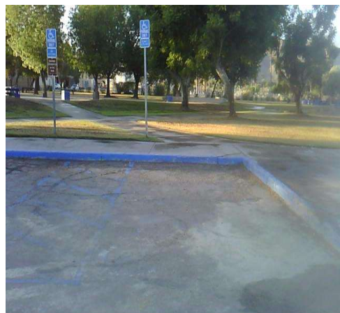
Parking Lot , Parking Space : Vehicle Encroaches Into Path of Travel
