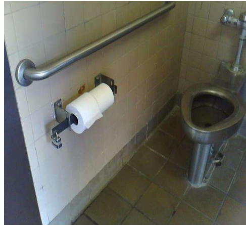
Restroom , Toilet Compartment : Toilet Paper Dispenser Distance From Seat
