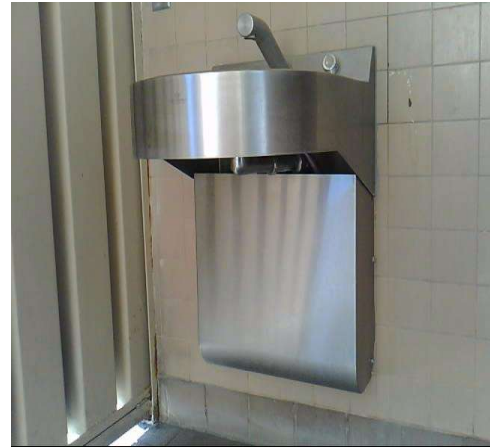
Restroom : Toe Clearance
