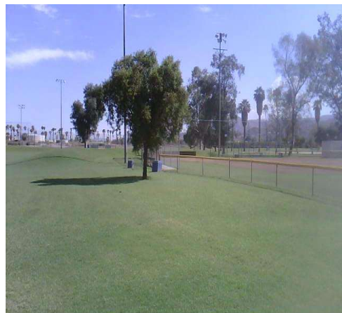
Path Of Travel , Walking Surfaces : Noncompliant Surface
