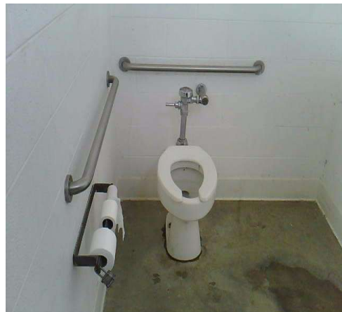
Restroom , Grab Bars : Distance from Front Edge of Toilet to Front of Grab Bar
