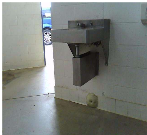
Restroom , Lavatory : Lavatory Pipes Not Wrapped
