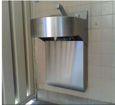
Restroom , Lavatory : Lavatory Pipes Not Wrapped
