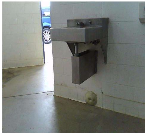
Restroom , Lavatory : Lavatory - Supply Lines not wrapped
