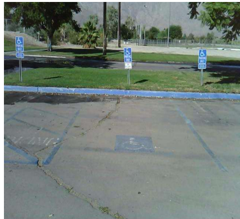
Parking Lot , Parking Space : Outline is Faded, Damaged or Missing
