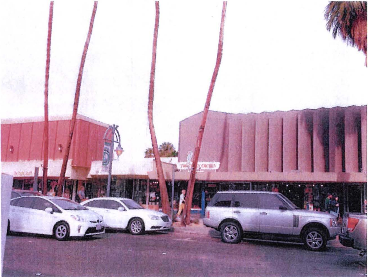
Photo 3. Palm Canyon Drive, looking east towards Building B (South Twin Building) and Building C (Bank of America Building), May 2014
