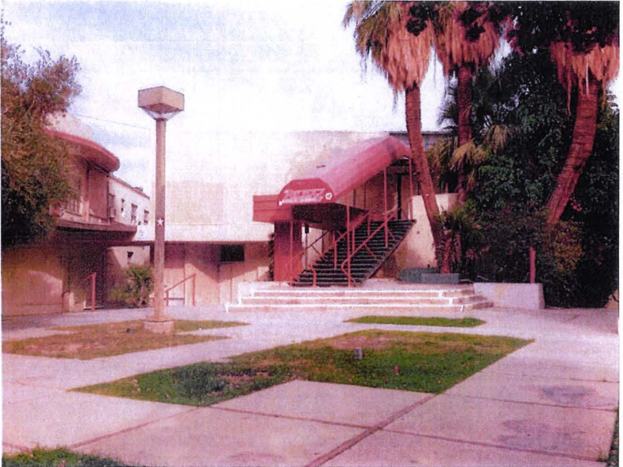
Photo 5. In the courtyard, looking east towards Building D (Town & Country Restaurant), May 2014
