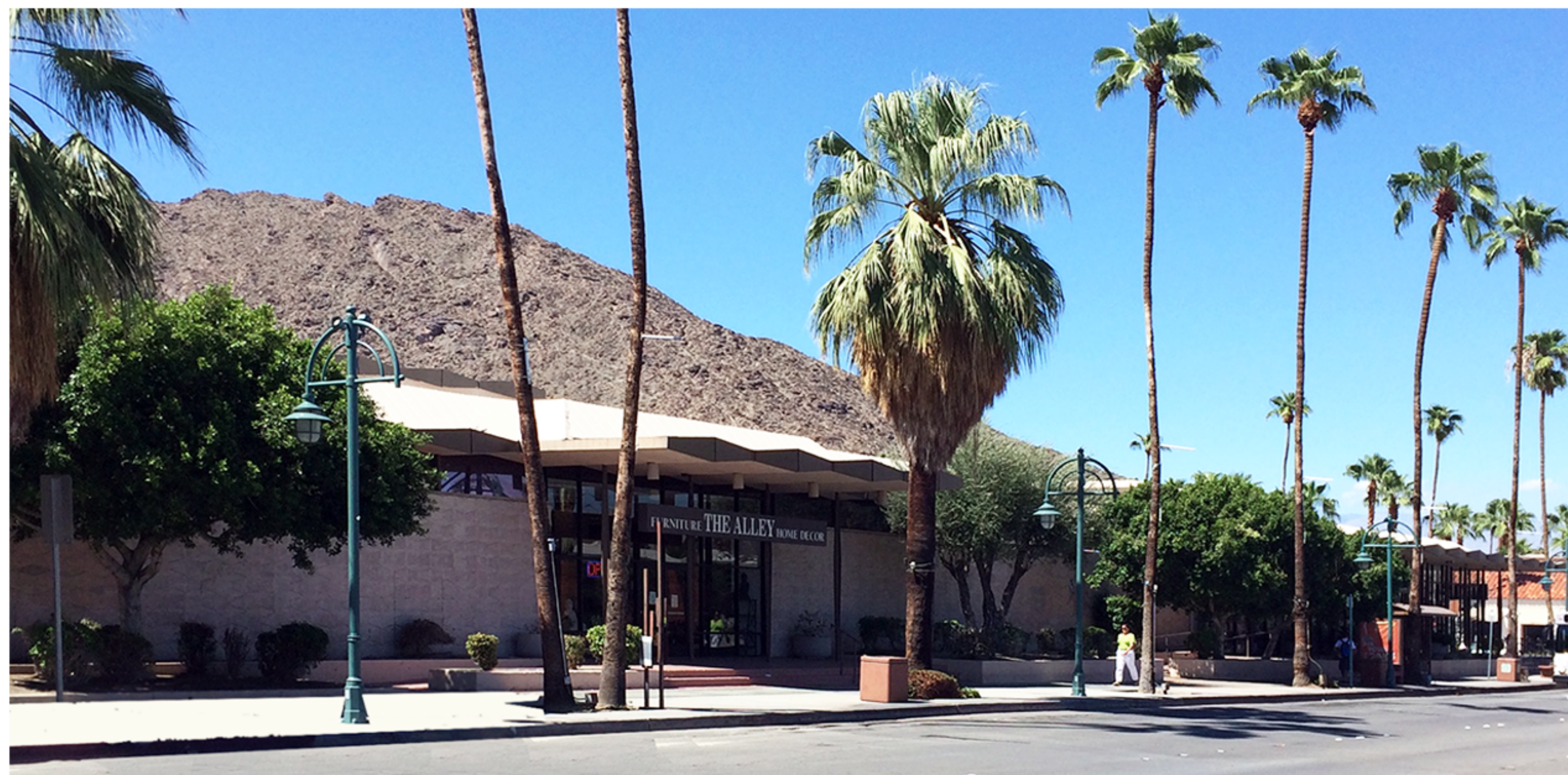
EXISTING IMAGE OF SOUTH EAST CORNER
