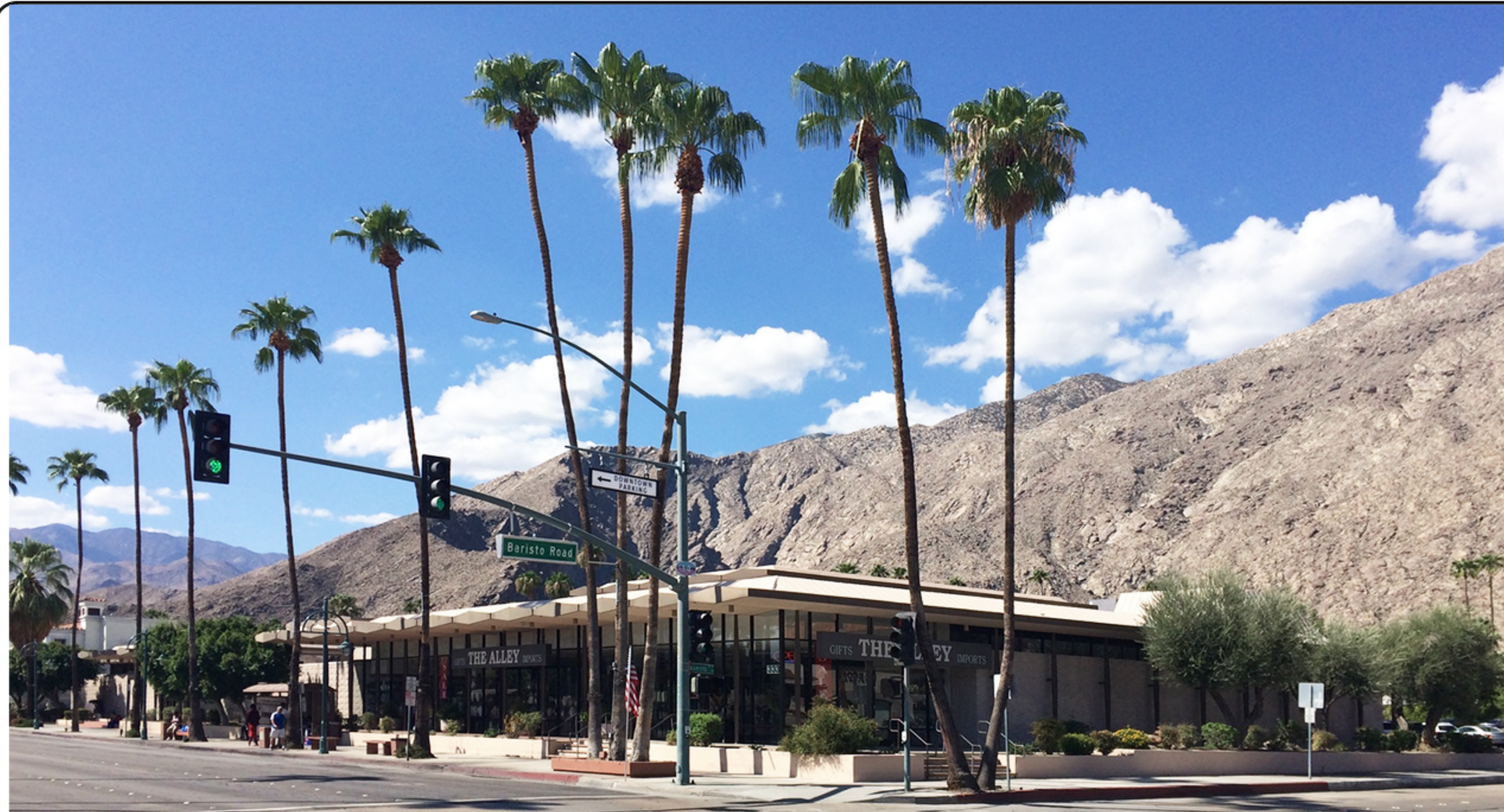
EXISTING IMAGE OF NORTH EAST CORNER
