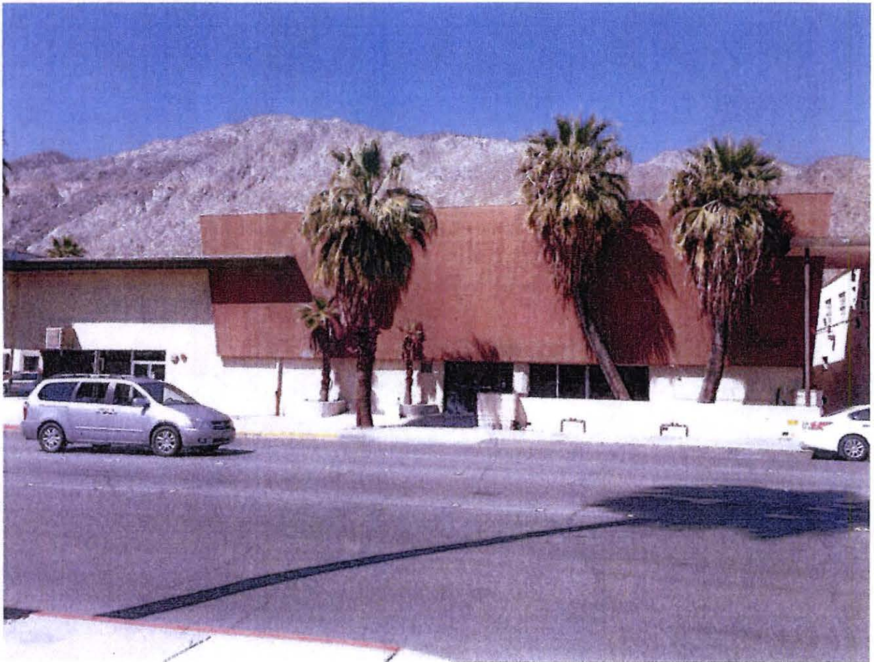
Photo 4. Indian Canyon Drive, looking west towards Building D (with a portion of Building A to the north), May 2014
