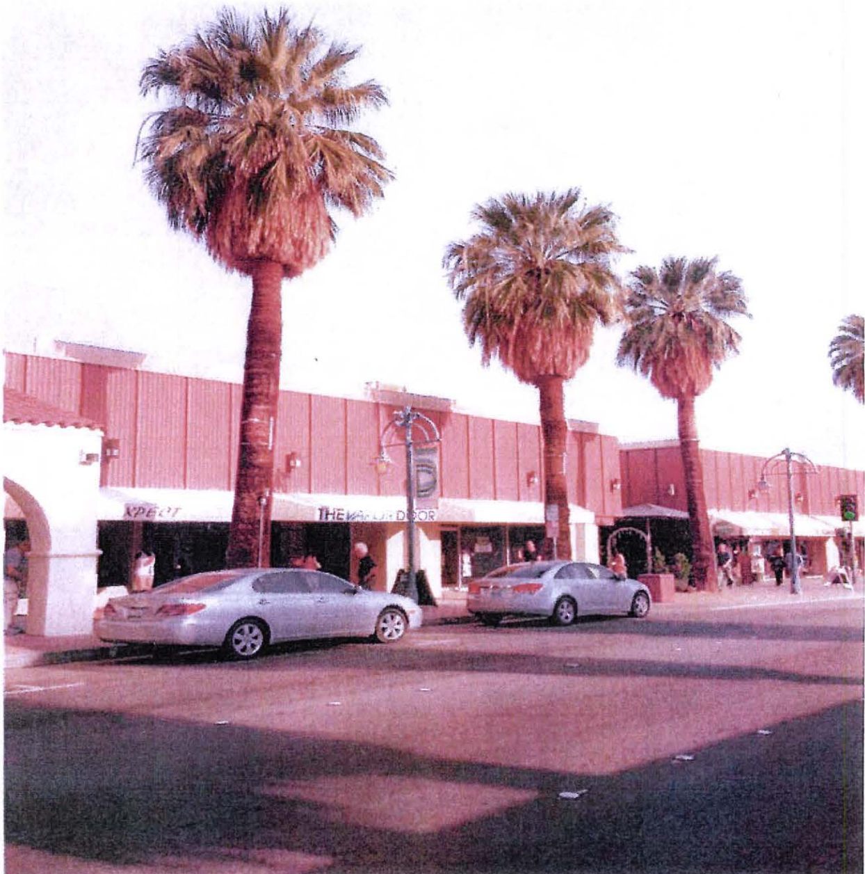
Photo 1. Palm Canyon Drive, looking South, Building A (Twin Building North) in foreground, Building B (Twin Building South in Background), May 2014
