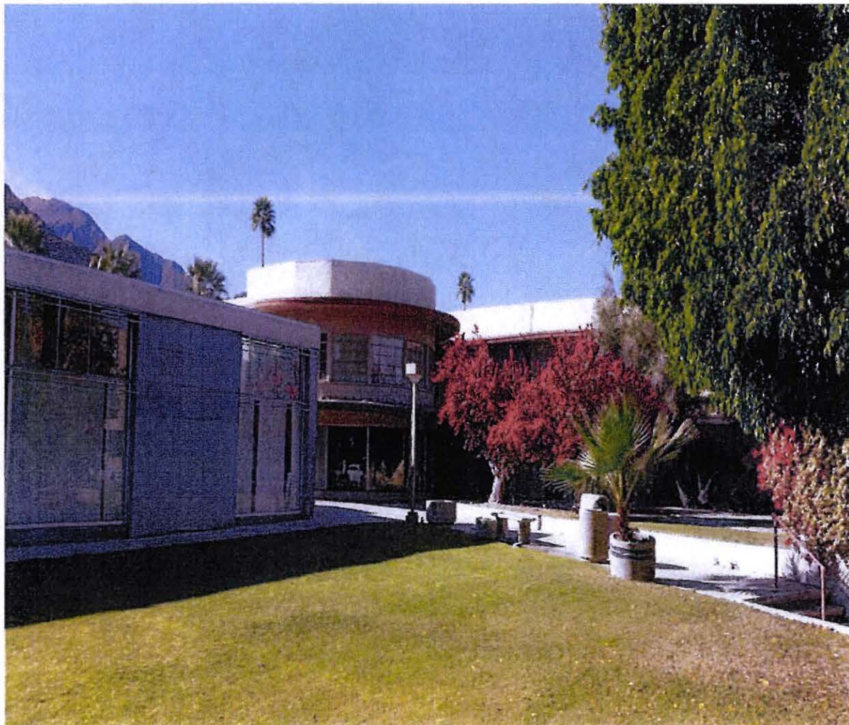
Photo 10. In the courtyard looking northwest toward Building E with Building A in background, March 2015
