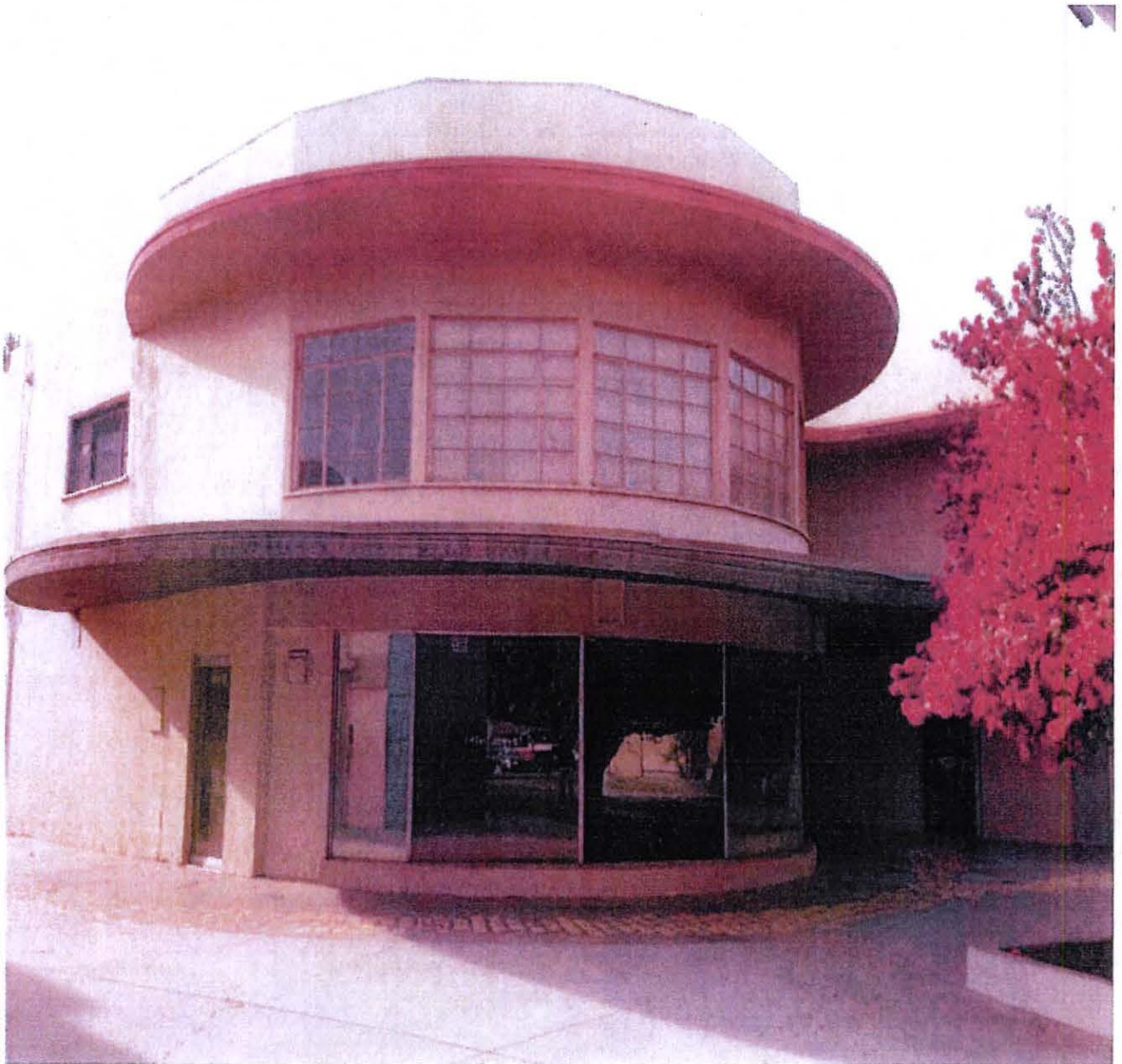
Photo 9. In the courtyard looking northwest toward Building A (Twin Building North), May 2014
