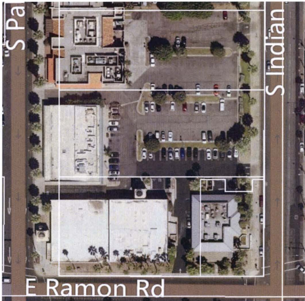
Aerial View of the South Palm Canyon Site
