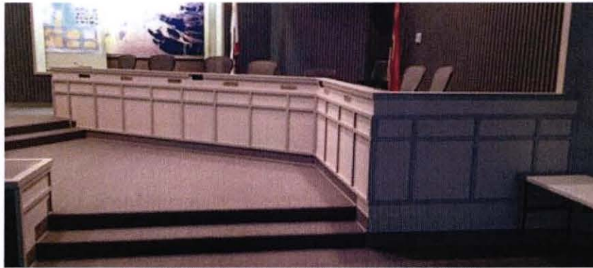
CLOSE UP VIEW OF CURRENT DAIS FROM 1984 RENOVATION
