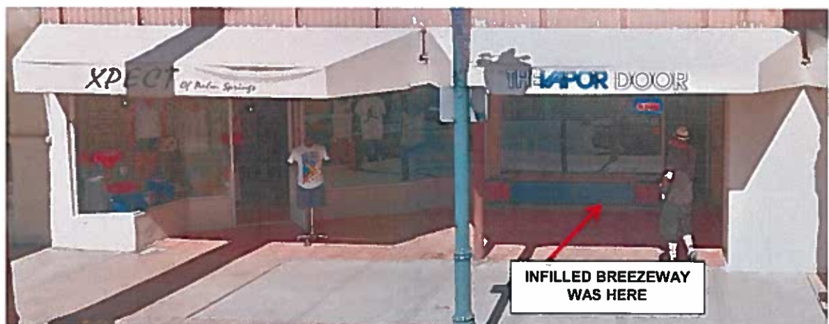
NOTE ANGLED STOREFRONT AT LEFT; TENANT SPACE AT THE RIGHT IS INFILL OF AN ORIGINAL PASEO OR "BREEZEWAY".
