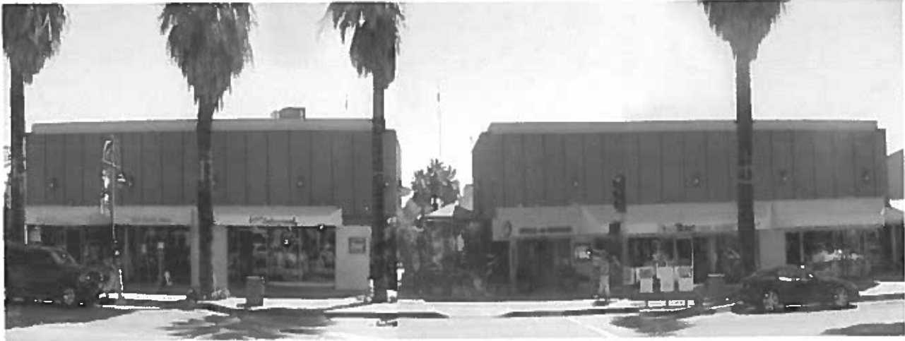
Current image of the Twin Buildings at 156-174 North Palm Canyon Drive. The passage to the Courtyard is partially blocked by an outdoor seating area. Palm Springs has no other examples of this kind of pairing.
