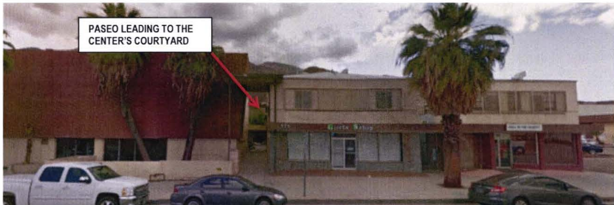
VIEW SHOWING THE 167 BUILDING, THE PASEO TO THE COURTYARD, AND THE 171 AND 181 BUILDINGS
