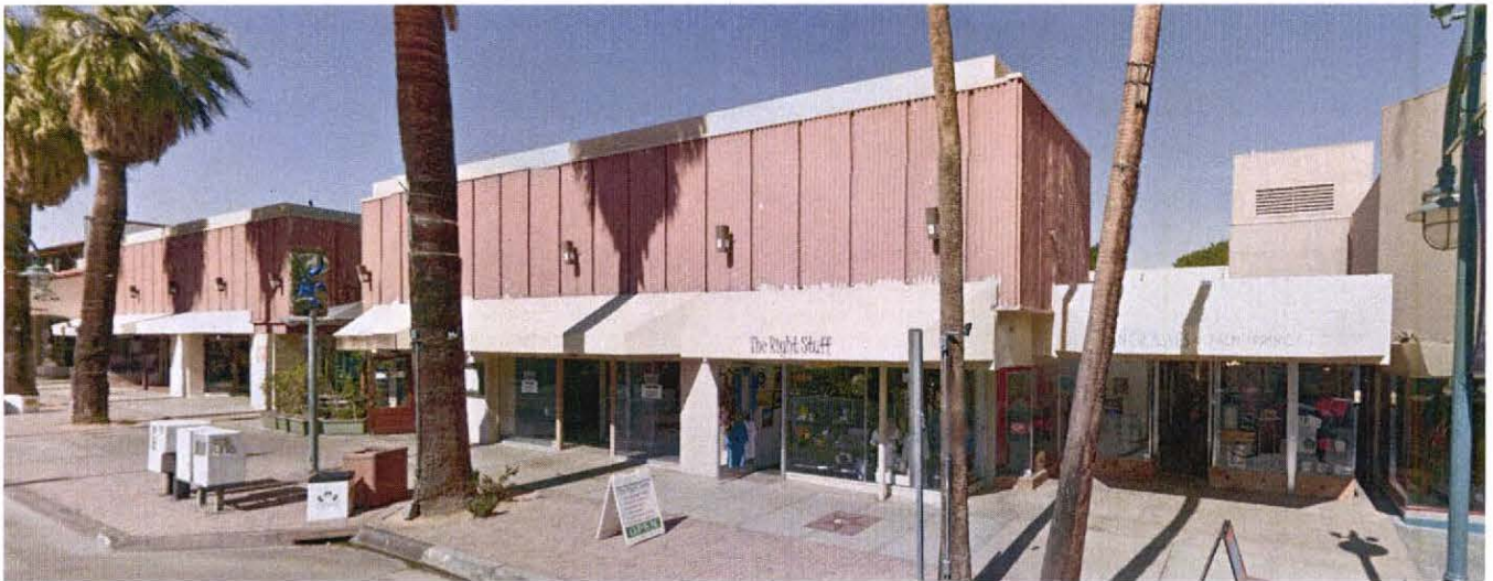
THE MATCHING FACADES OF THE 156-166 BUILDING (FOREGROUND) AND THE 170-174 BUILDING (FAR LEFT)
