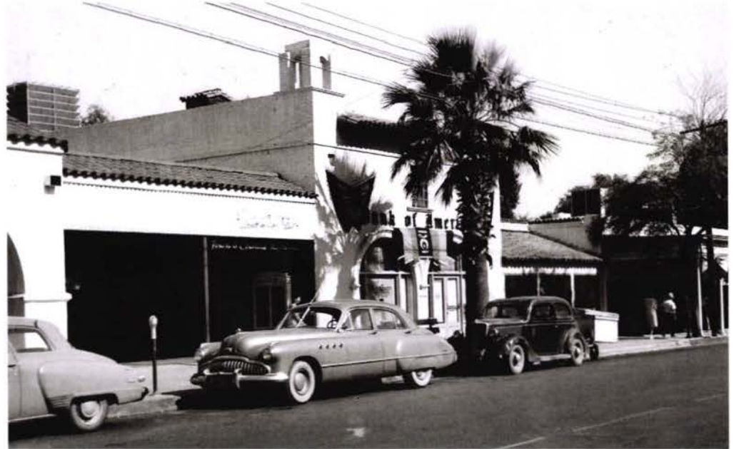
Town & Country Restaurant Entrance North Palm Canyon Drive 1948
