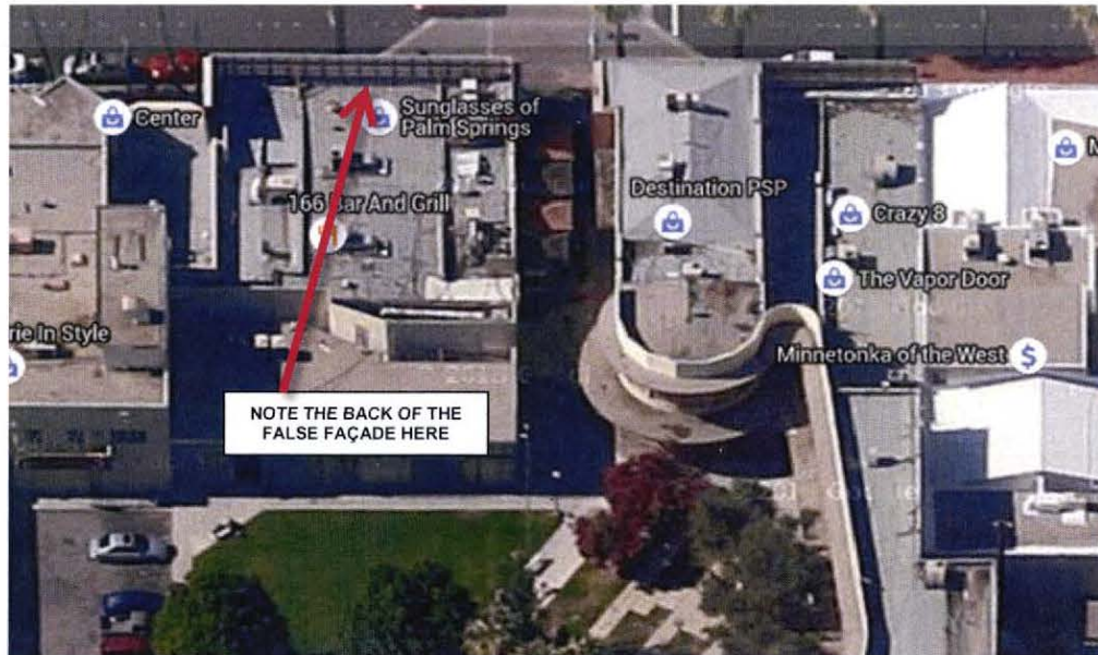
THE AERIAL PHOTO ABOVE SHOWS THE FALSE FAÇADE OF THE 156-166 BUILDING (CENTER LEFT) AND THREE ROOF AREAS OF DIFFERING SLOPES SEPARATED BY LOW PARAPET WALLS. THE 170 BUILDING, WITH THE SEMI-CIRCULAR EAST FAÇADE IS THE ONLY TWO-STORY PORTION OF THE 156 - 174 BUILDINGS.
