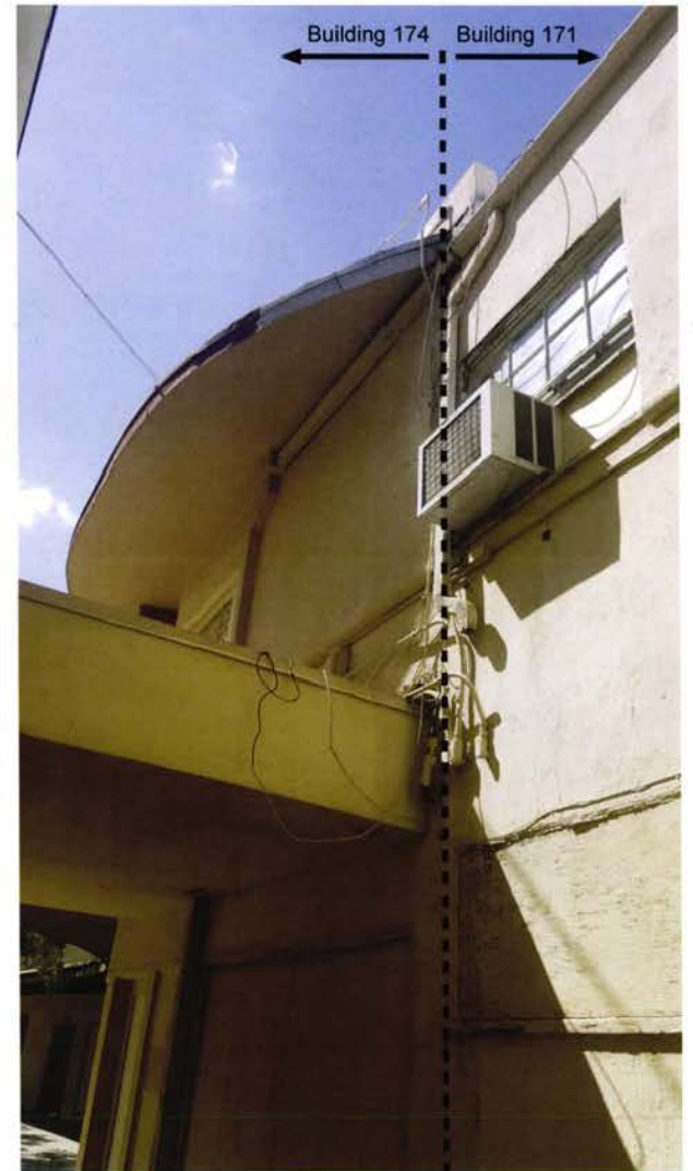
Connection Point of Building 171 and 174 2016
