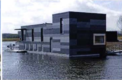
EQUITONE PANEL FACADE
