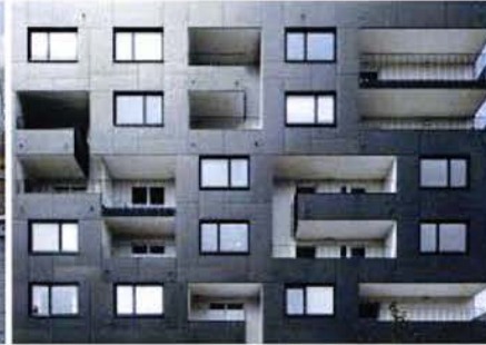
EQUITONE PANEL FACADE
