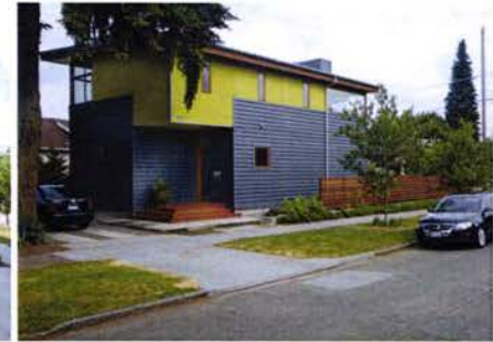
BOXED CORRUGATED GRAY METAL SIDING
