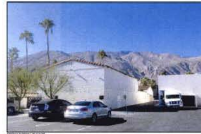
EXISTING PARKING LOT FACADE
