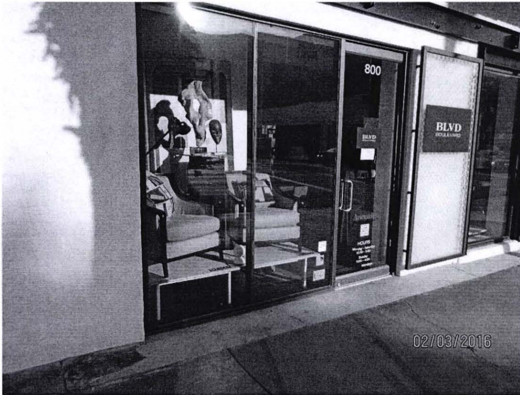
The picture above is an example of an existing storefront in the El Paseo Building facing North Palm Canyon Drive with the proposed treatment. In this case the glass is affixed to an aluminum frame.
