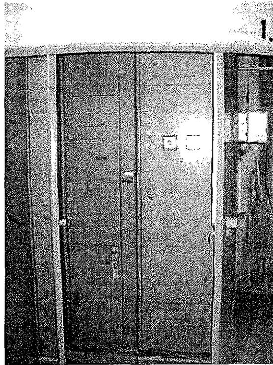
**Figure 10 – Secondary Gallery “Upper” Level Motor Control Center**
