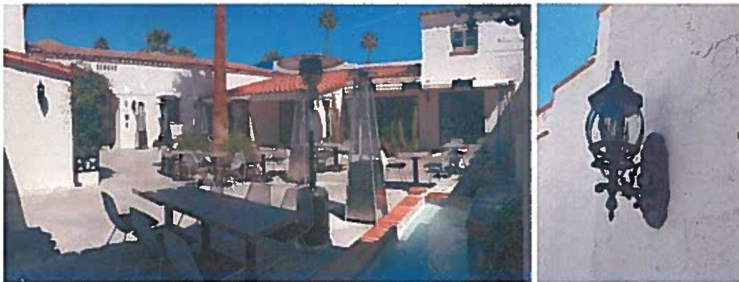
VIEW LOOKING TOWARD THE NORTHWEST CORNER AND EXAMPLE OF EXISTING WALL SCONCE (NOT ORIGINAL)
