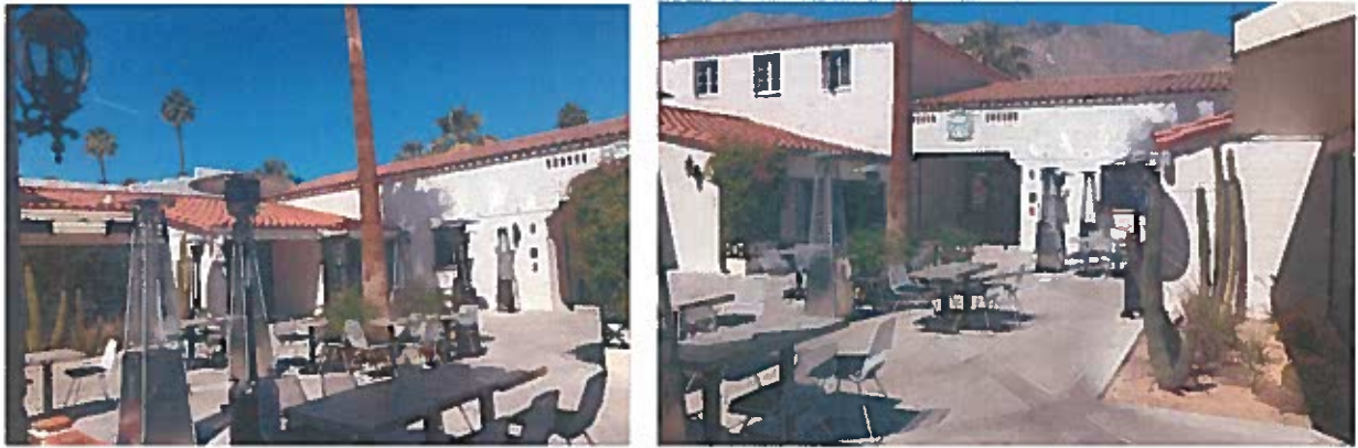
VIEWS WITHIN THE COURTYARD LOOKING TOWARD THE WEST
