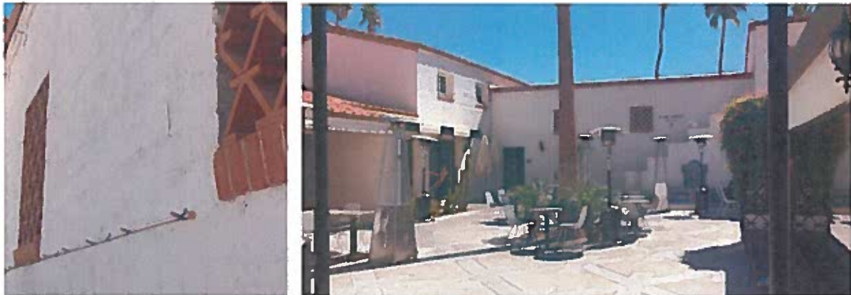
VIEW LOOKING EAST
