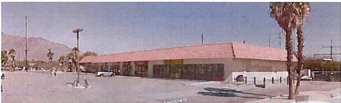
SOSSA'S CENTER (PROPOSED MARKET IS IN THE EASTERMOST TENANT SPACE)
