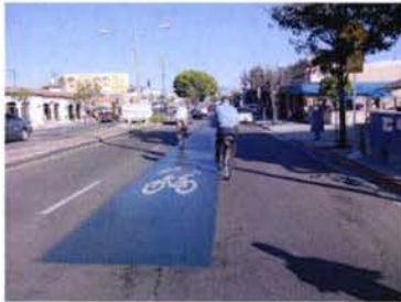
FIGURE 15 Brookline, MA Sharrow markings
