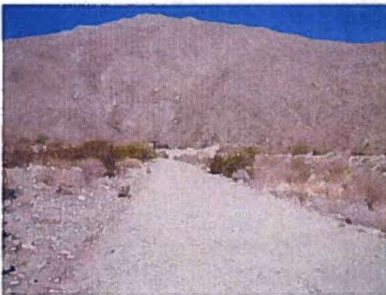
On the south side looking west towards the spillway
