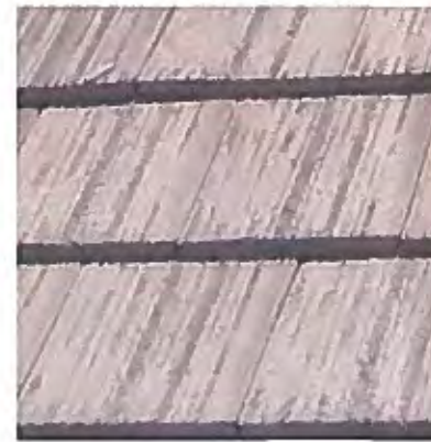
6 [EF-8] EXISTING ROOF TILES
