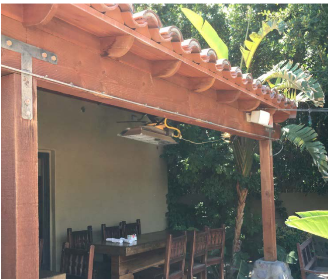
Misters at the El Mirasol building
