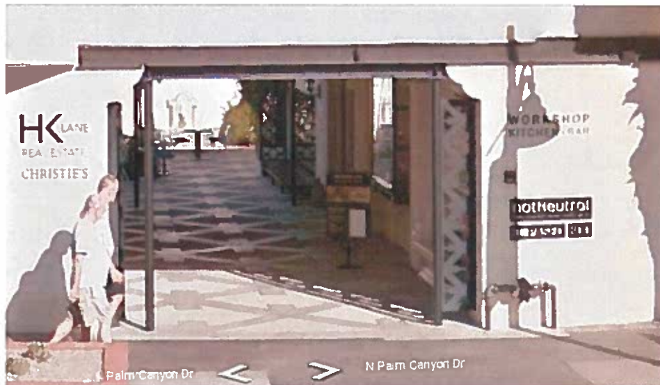
VIEW FROM PALM CANYON LOOKING THROUGH THE PASEO INTO THE COURTYARD – PAVING PATTERN IS NOT ORIGINAL
