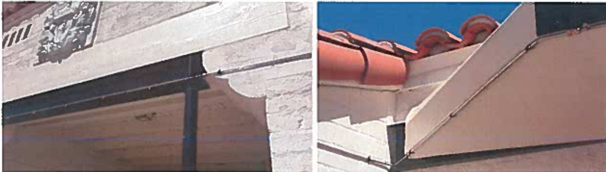
DETAIL ABOVE THE PASEO LEADING TO PALM CANYON AND AT NORTHWEST CORNER SHOWING NEW MISTING PIPING
