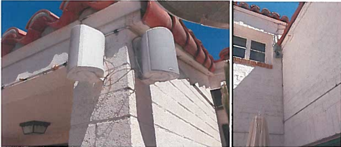
DETAIL ALONG THE NORTH WALL OF THE COURTYARD AND THE NORTHEAST CORNER SHOWING NEW MISTING PIPING
