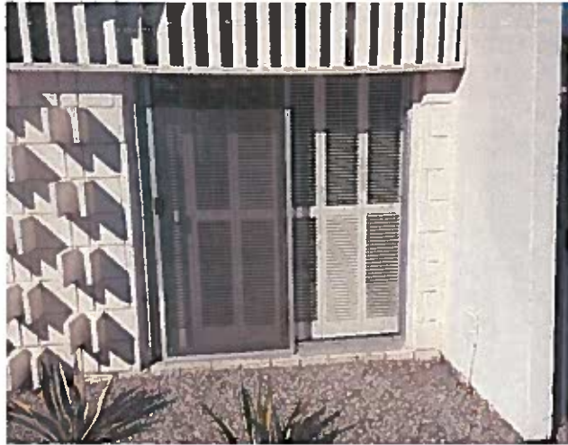
Block Removed Sliding Door Added
