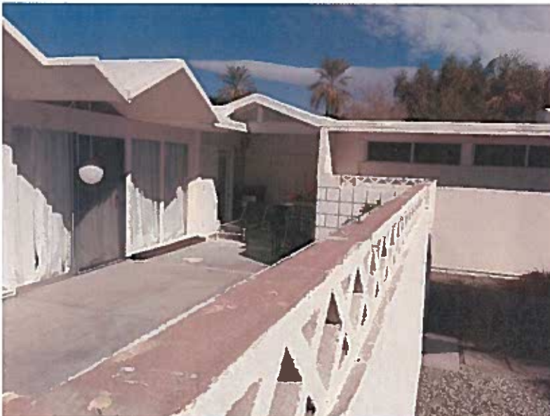
Roof Added Over Patio
