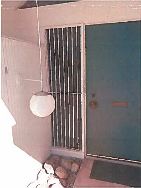
Security Bars Added To Jalousie Windows
