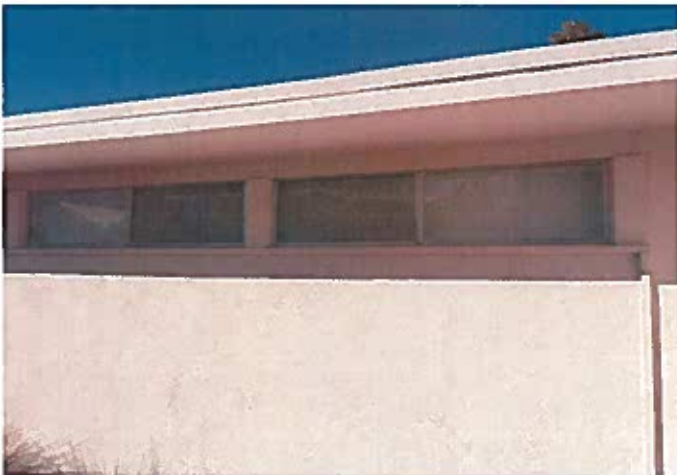
Fixed Windows Made Operative
