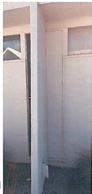
Jalousie Bedroom Window Removed
