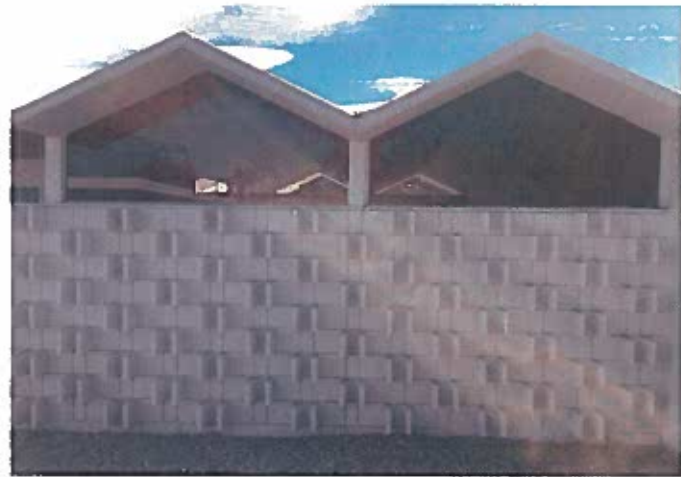
Clerestory Windows Reglazed Without Mullions
