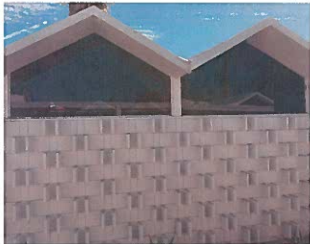
Clerestory Windows Reglazed Without Mullions
