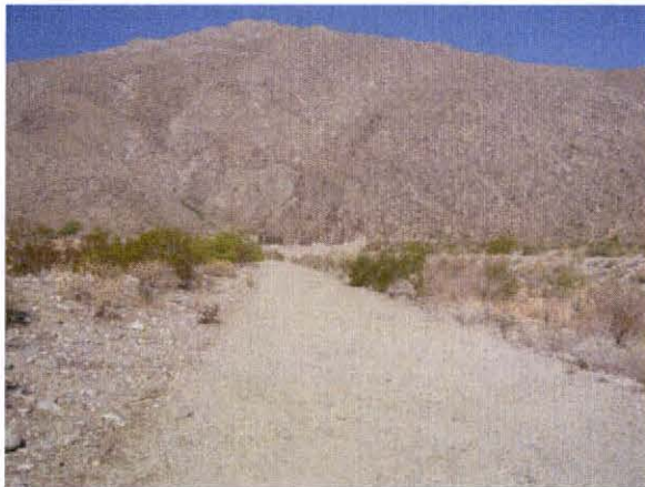
On the south side looking west towards the spillway
