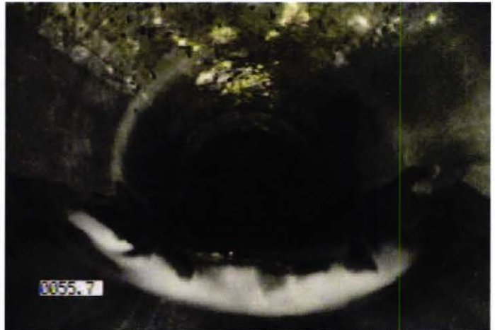
DV - Brick Deformed Vertically @ 55.7 ft.
