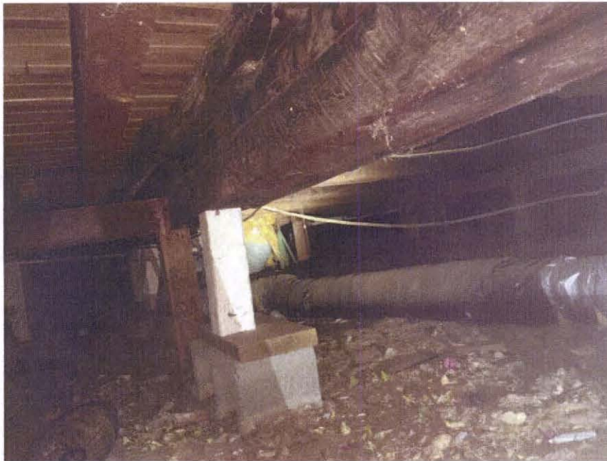
Figure 2: Existing crawlspace, interior support
