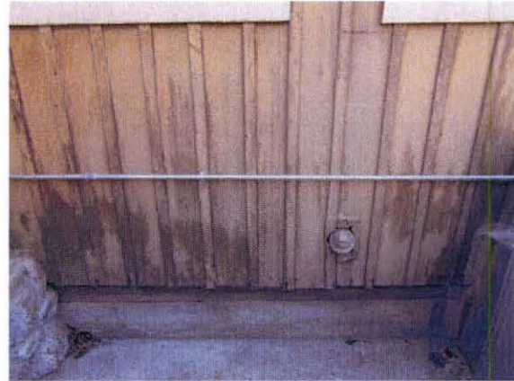
Board and batten siding at west elevation of Kitchen.
