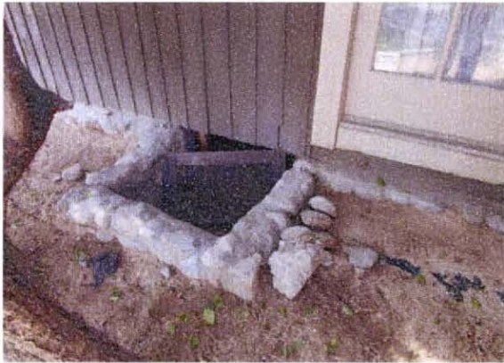
Crawlspace entry at east elevation.
