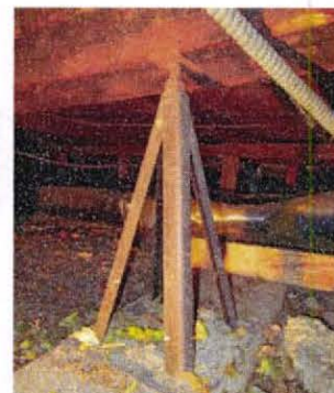
Metal tripod support at crawlspace.
