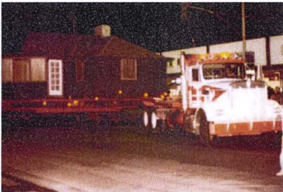
Relocation in progress, 1979. Note enclosed porch at left of image. (Photo courtesy: Palm Springs Historical Society)
