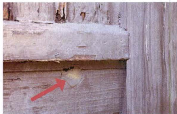
Prior epoxy repair at west elevation.
