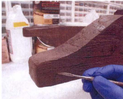
10. Epoxy fill being tooled to mimic wood grain.
