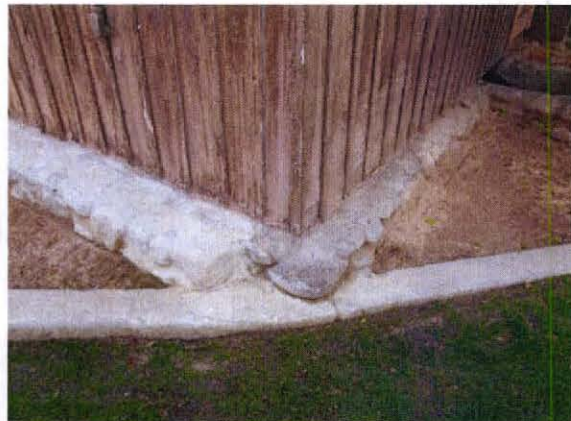
Foundation wall stone detail at southeast corner.
