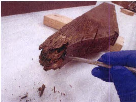
3. Mechanical removal of decayed wood.
