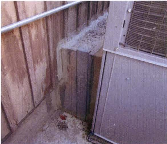
Modified siding at west elevation for HVAC equipment.
