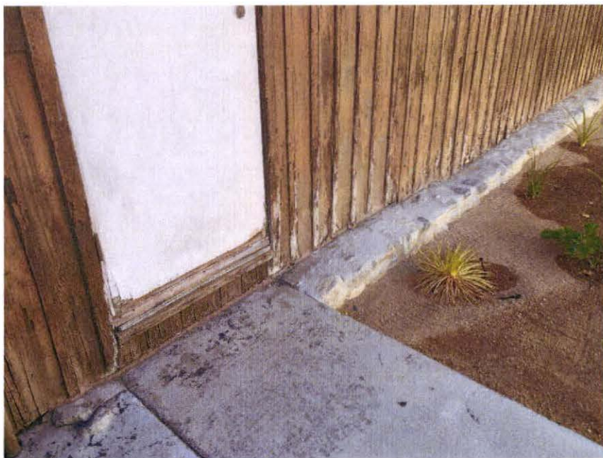
Figure 7: Existing wall with board-and-batten siding
