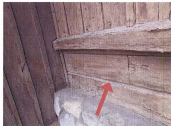
Chamfered edge detailing still visible at cross ties at east elevation.
