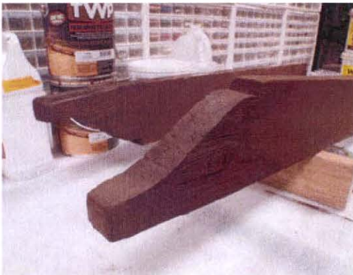
9. Epoxy fill being shaped to match rafter tail end.
