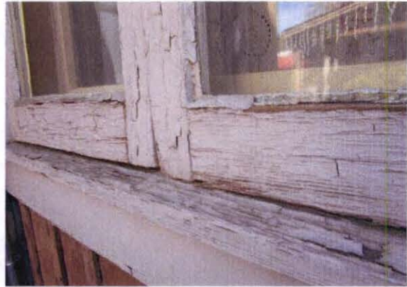
Typical condition at base of windows.
