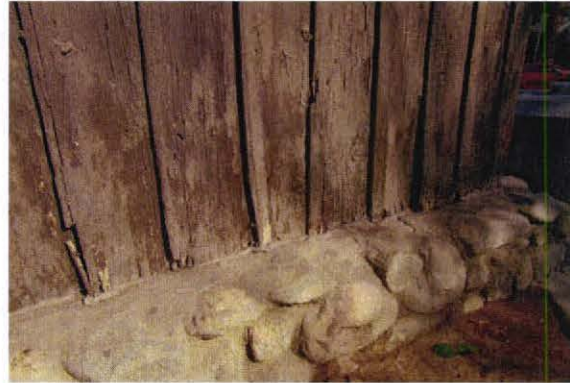
Board and batten siding at south elevation of Bedroom.
