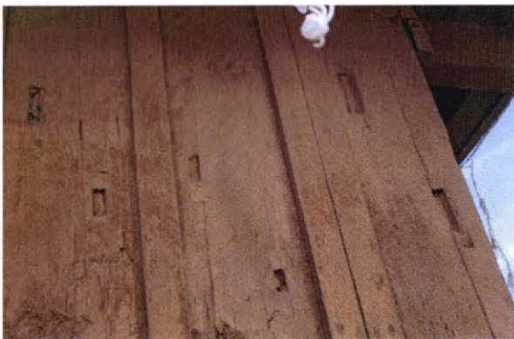
Cross ties at east elevation. Note mortises and other surface features.
