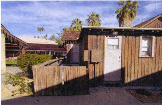
Mechanical area at southwest corner.
