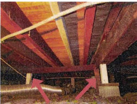
View in crawlspace looking north. Note beam post supports.
