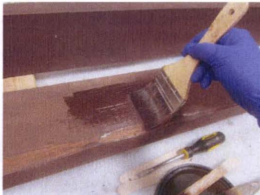
16. Application of dye stain. (Not applicable for painted finish)
