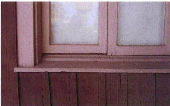
Modified sash at Bedroom window, north elevation
