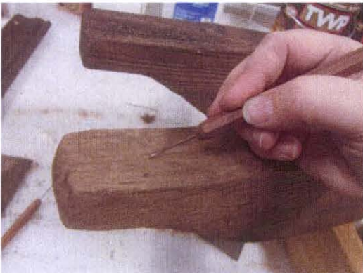
15. Additional tooling of epoxy fill surface.
