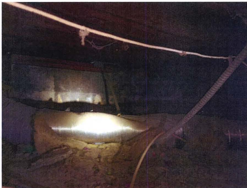
Figure 3: Existing crawlspace, perimeter concrete footing
