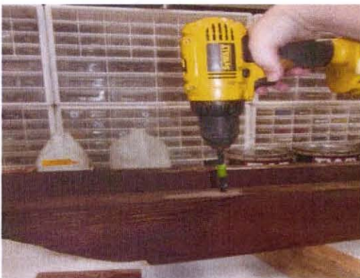
11. Drilling hole to for borate rod.
