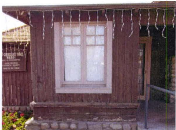
Replaced window at north elevation of Bathroom.
