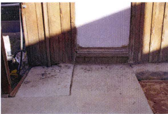
Concrete slab Kitchen door entrance.
