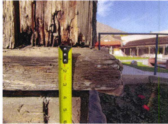
Belt course at northeast corner. Note bottom 1/2-inch removed.
