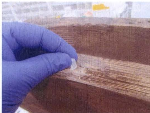
12. Inserting borate rod. Set 1/4-inch below surface.
