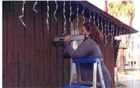
Resistograph testing at east facade.
