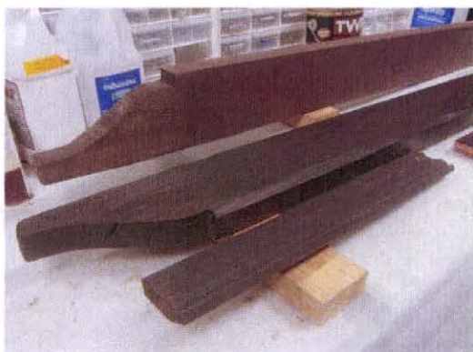
19. Completed rafter repair.
