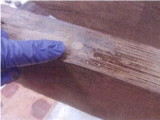
13. Completed epoxy fill at borate rod.
