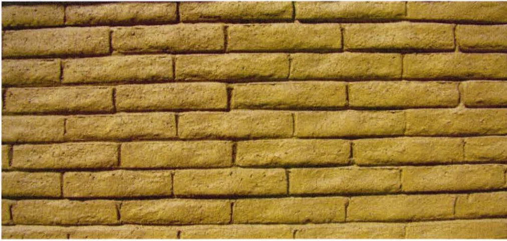
Detail of mortared concrete slumpstone block, a building material ideally suited to the harsh desert environment.
