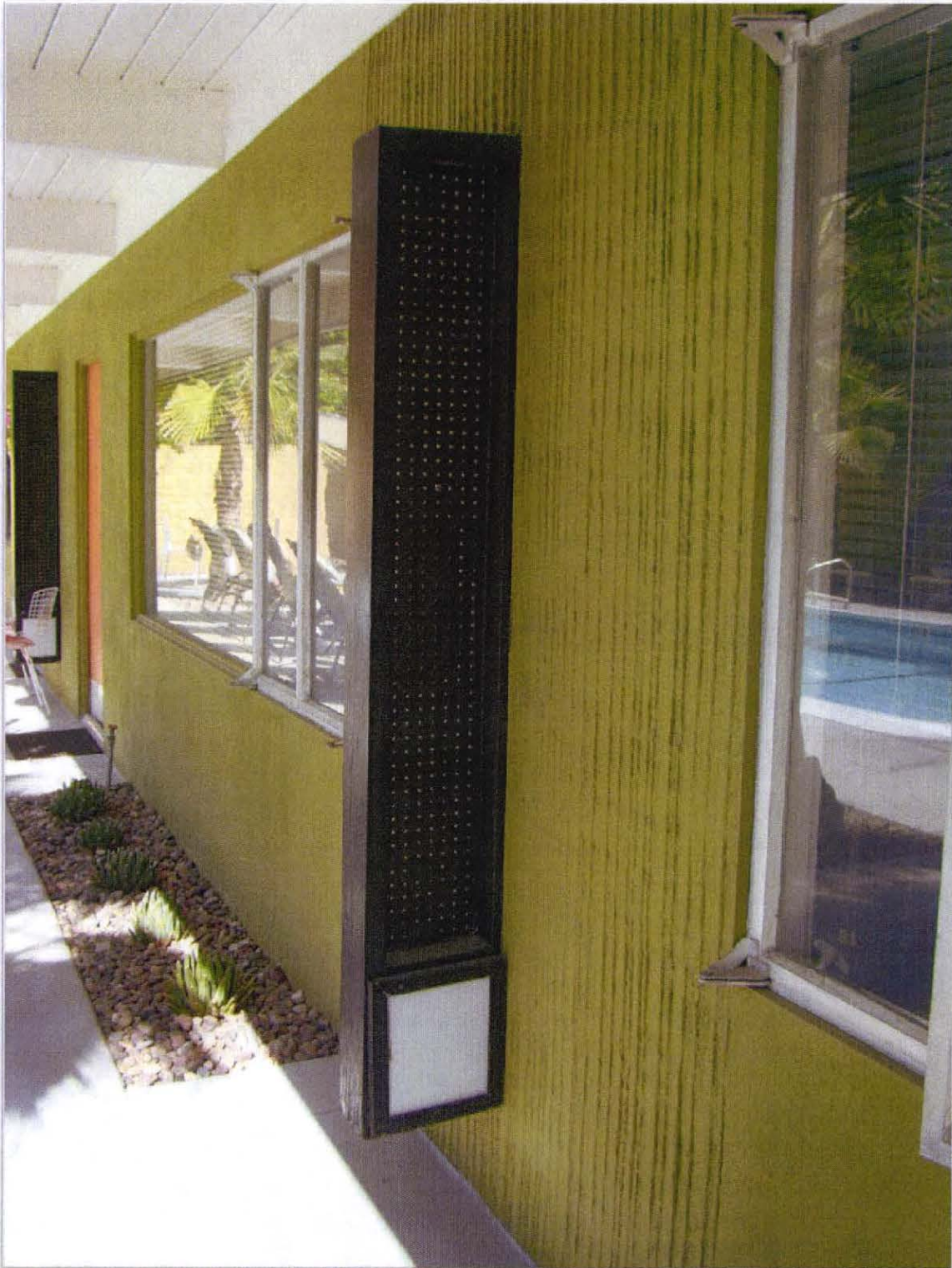
Shown here are multiple architectural details: (1) deep eave with wood tongue-in-groove and horizontal structural wood support beams, (2) vertically raked concrete stucco walls, (3) casement windows, (4) planter flush with the concrete flatwork, and (5) a custom-designed "floating" vertical lighting fixture of wood and pegboard.
