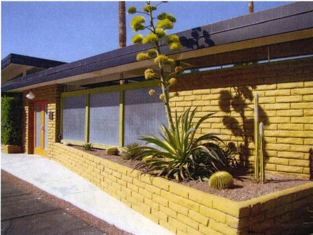
A triangular planter (about 2-feet high) constructed of concrete slumpstone block extends outward from the front façade to create visual interest and emphasize the overall horizontality of the structure. The planter's triangular shape cleverly mimics the shed roof (seen far left).
