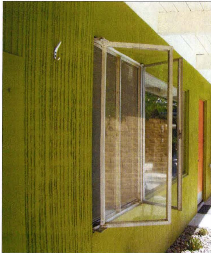
Casement window, vertically raked concrete stucco, flush planter, horizontal support beams and tongue-in-groove ceiling in deep eave.
