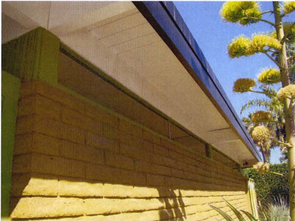
Clerestory window under deep eave (east side of Unit #1).
