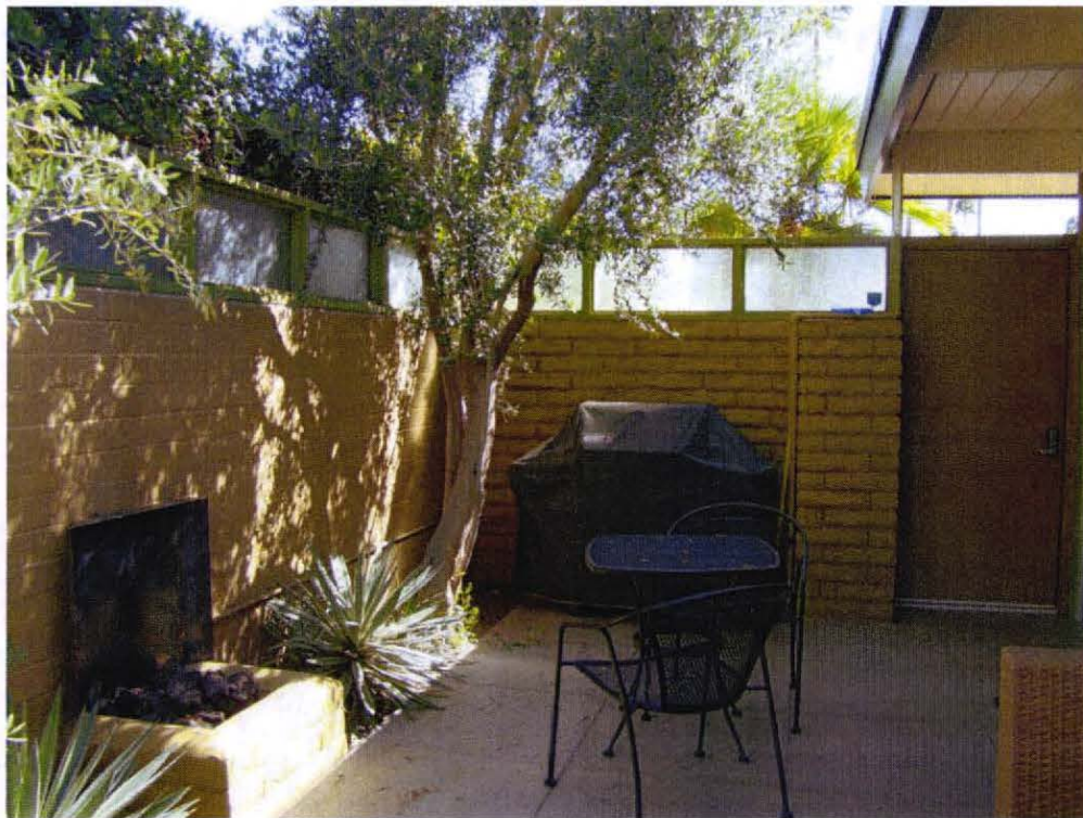
Enclosed patio showing later door and wood-framed glass panels added for privacy and security. Not shown are original plywood doors which separate the individual patios.
