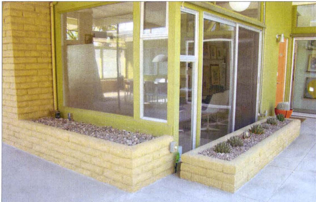
Small slumpstone planters are alternately either stand-alone or integrated into the structure. While these two planters are of roughly the same length and width, they are of different heights to create visual interest. Installed plantings serve as a counterpoint to, and soften, the rectilinear modernist architecture. This photograph also shows modernist architecture's expansive use of glass intended to blur the transition between the indoors and outdoors.
