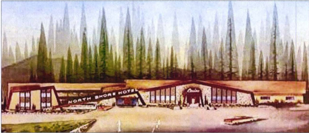
The North Shore Club Hotel in Crystal Bay (Lake Tahoe), Nevada was “rebuilt” in a modernist design by Howard Lapham in 1960.
