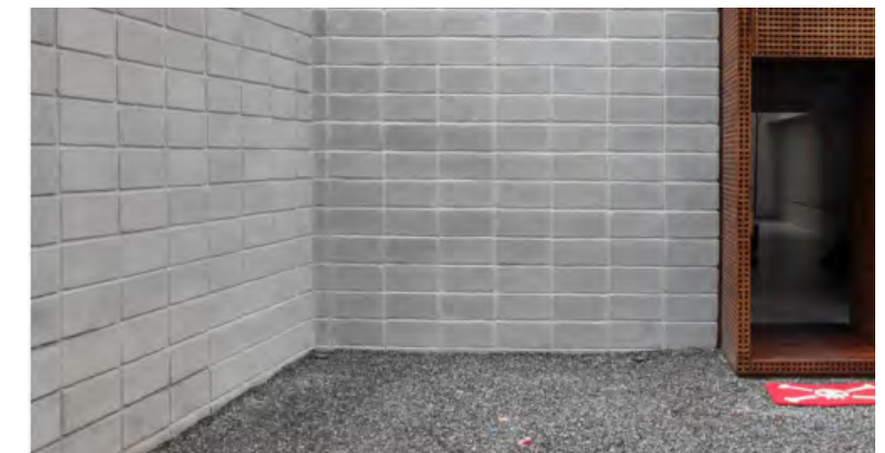
C.M.U. Block - Side Yard Walls
