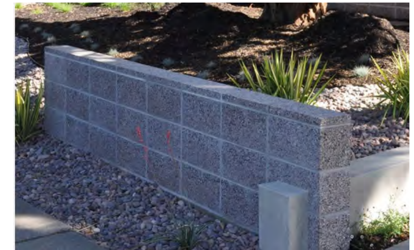
Burnished Block - Courtyards / Corner Lot Walls
