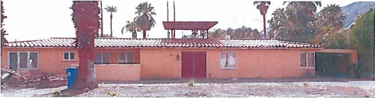
STREET VIEW OF SUBJECT PROPERTY
