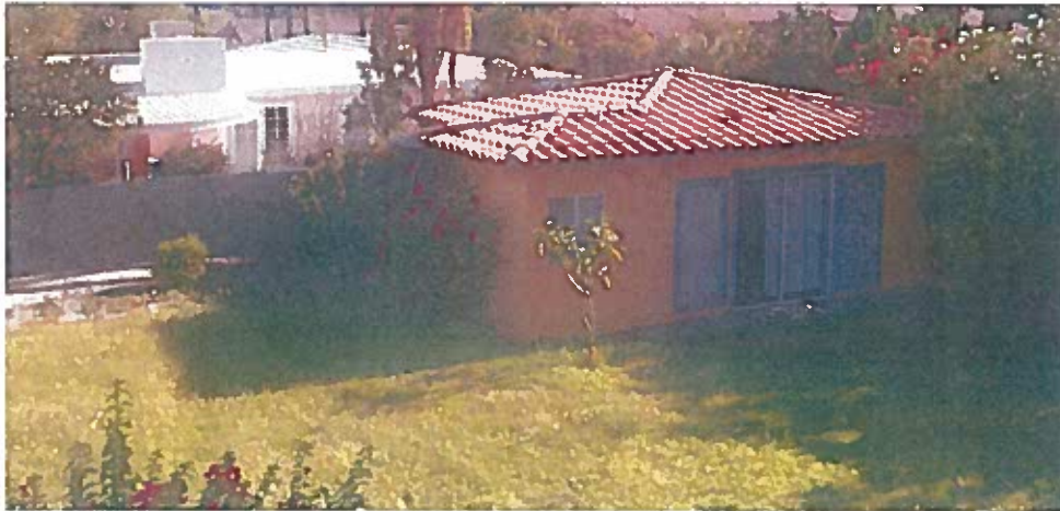
NON-PERMITTED CASITA IN BACK YARD
