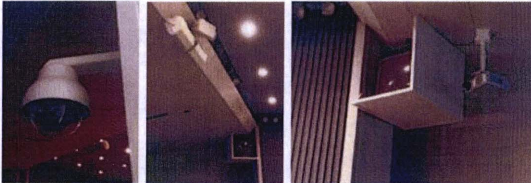
EXISTING CAMERAS, SPEAKERS, TV MONITORS AND PROJECTION EQUIPMENT WILL BE REMOVED AND REPLACED.
