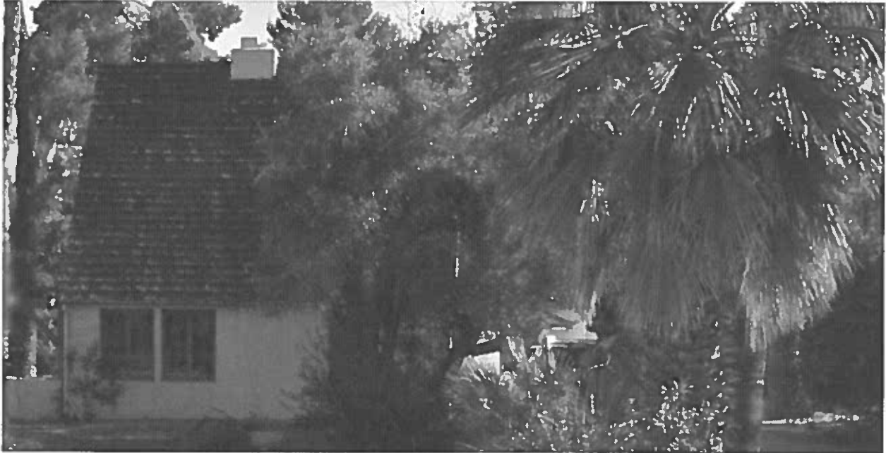
PARTIAL STREET VIEW OF 401 MERITO PLACE.
