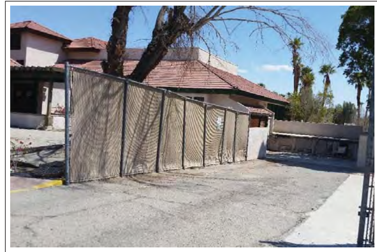
Looking east at service area at the southern section of the site
