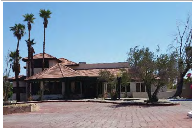
Looking east at restaurant building from entry driveway
