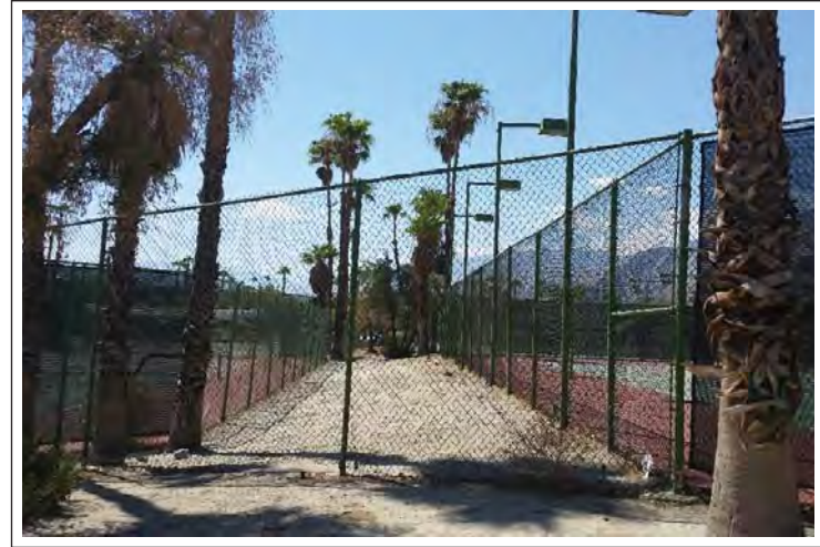
Looking south at tennis courts at the eastern section of the site
