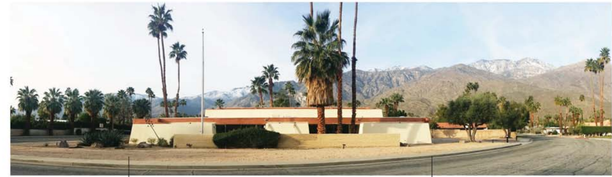
Existing Fire Station #4 from Marion Way
