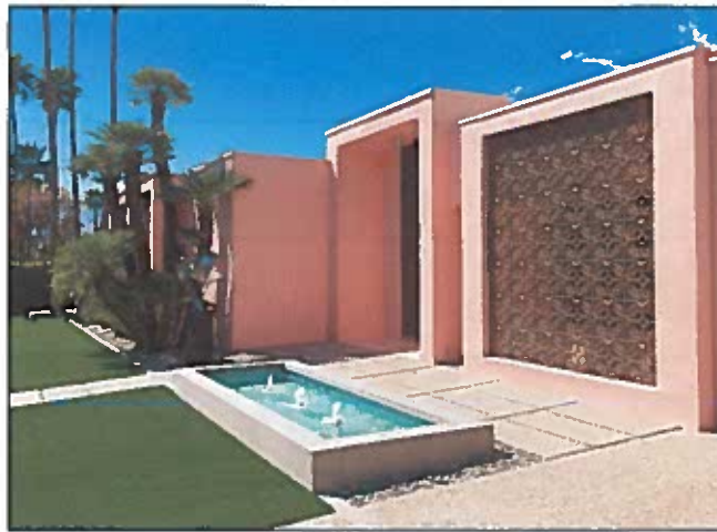
The 2016 addition of the front yard fountain compliments the rectilinear design of the residence.
