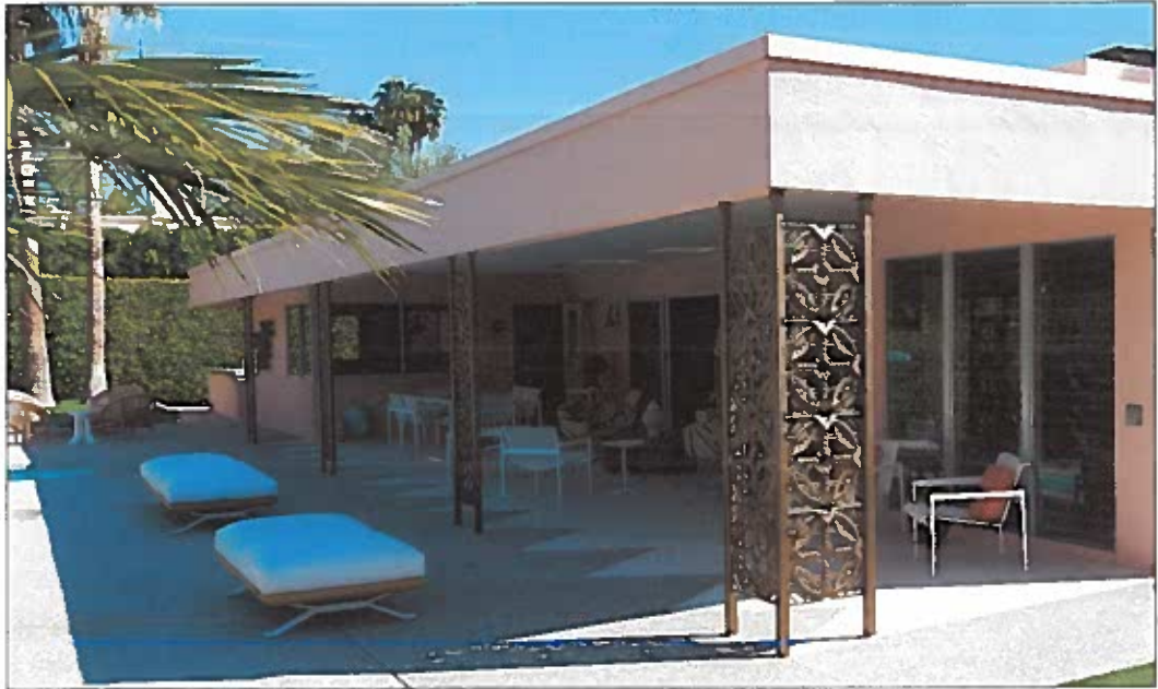
This image shows numerous features on the west side of the residence, including the shade created by the deep loggia, structural supports adorned with AGUs, and the sawtooth edge of the original terrazzo.
