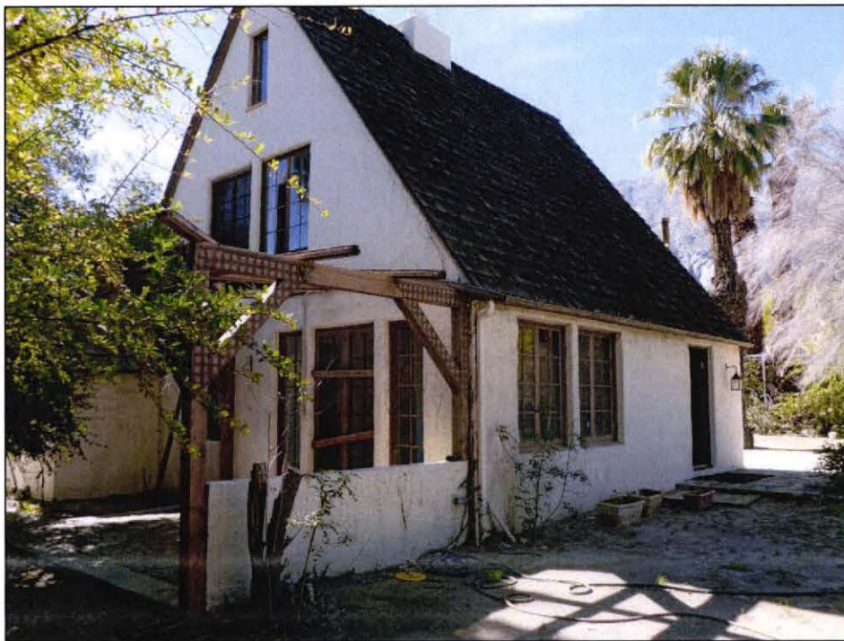
East and north façades, view to southwest.
