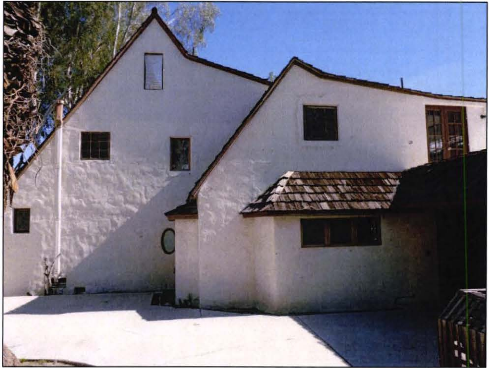
West façade, view to east.
