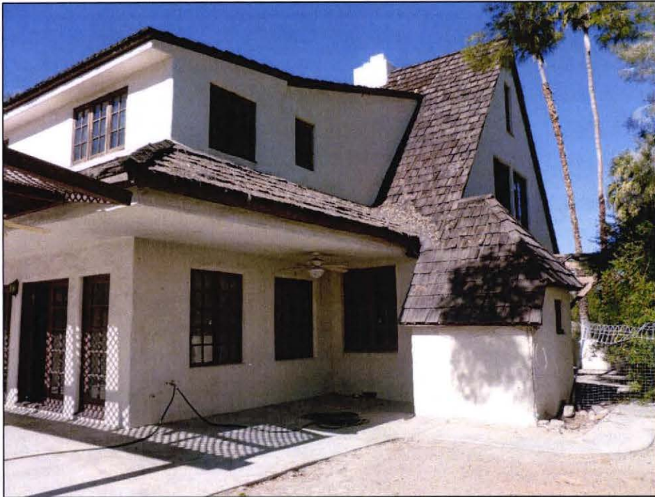
East façade, view to northwest.
