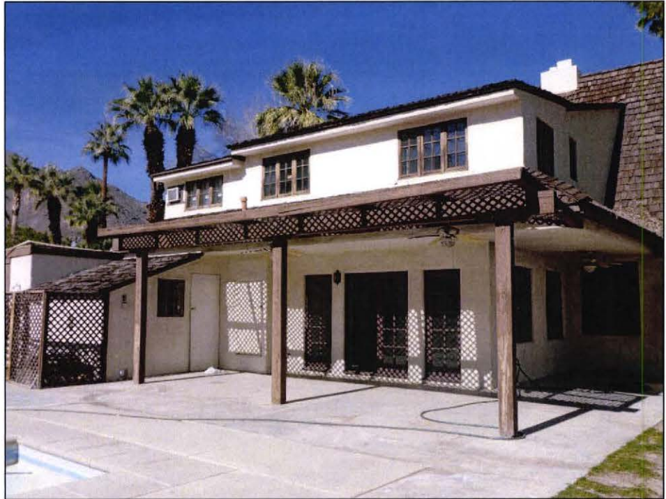
South façade, view to northwest.
