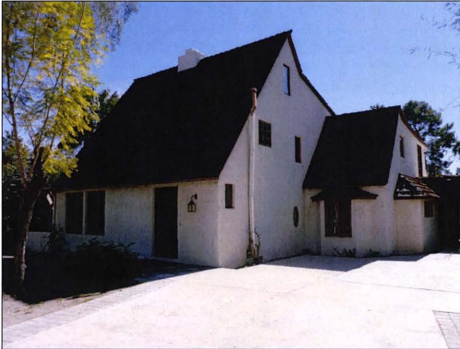
North and west façades, view to southeast.
