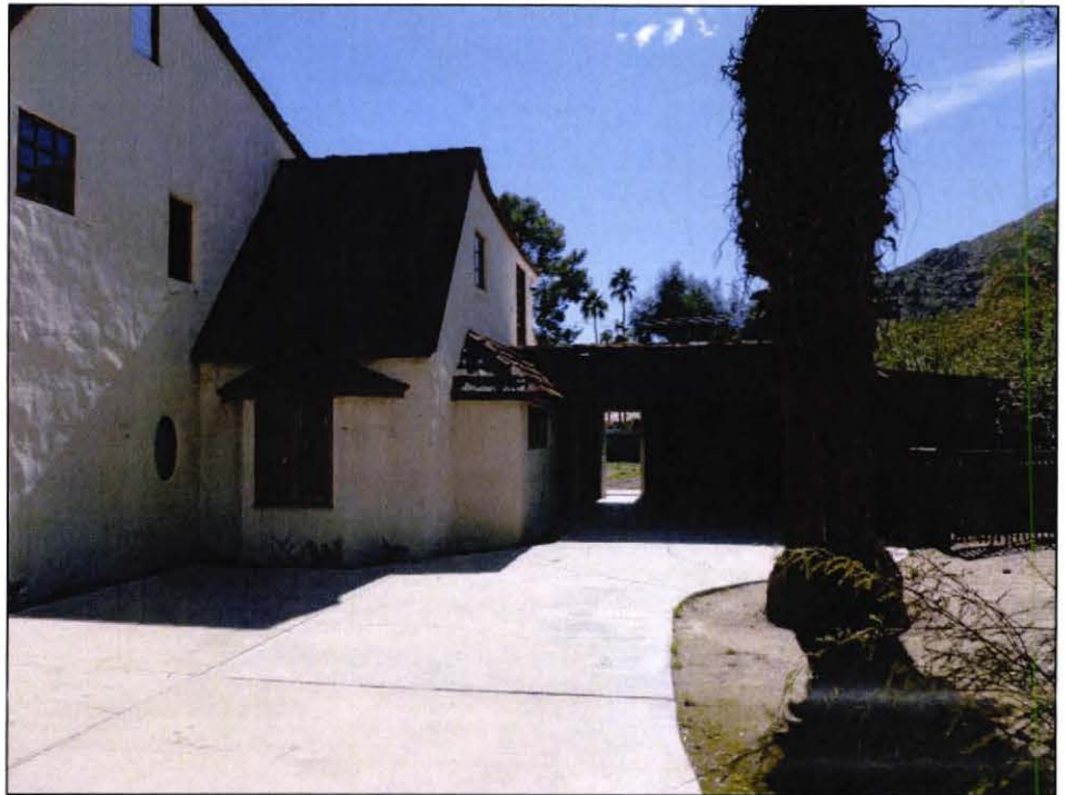
Attached carport at west façade, view to south.
