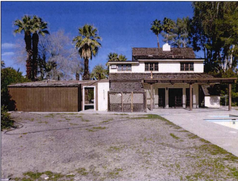
South façade, view to north.
