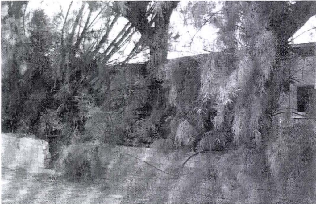
Figure G.1 Building "G"- Shed Building
