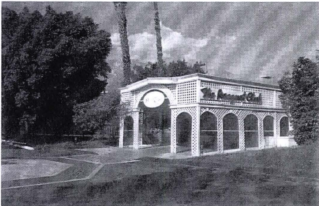
Figure A.6 Building "A"- Lobby/ Office Building
