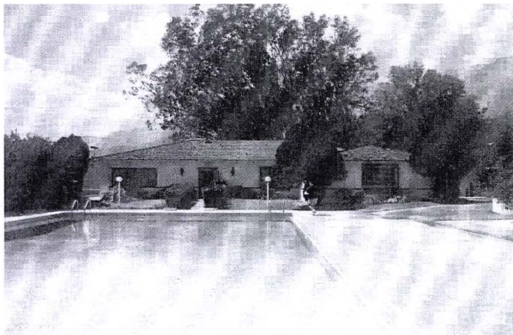
Figure D.1 Building "D"- Farrell House
