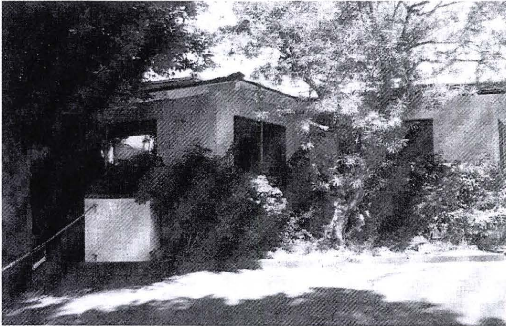
Figure A.5 Building "A"- Lobby/ Office Building
