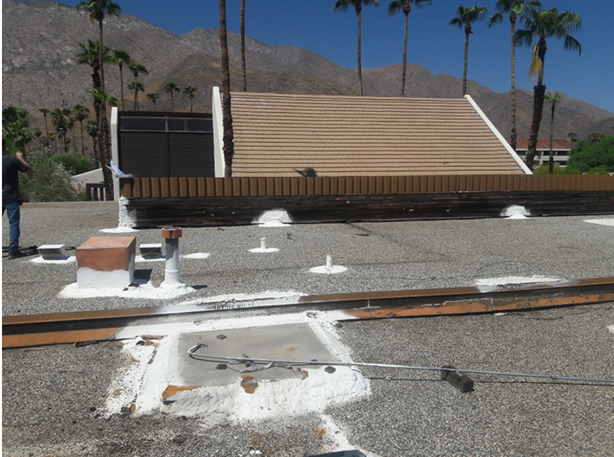
ROOF VIEW OF 650 E. TAHQUITZ CANYON WAY FACING WEST
