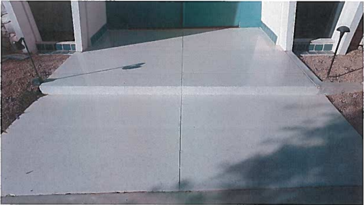
Terrazzo walkway to front door. Also note glazed turquoise tiles.
