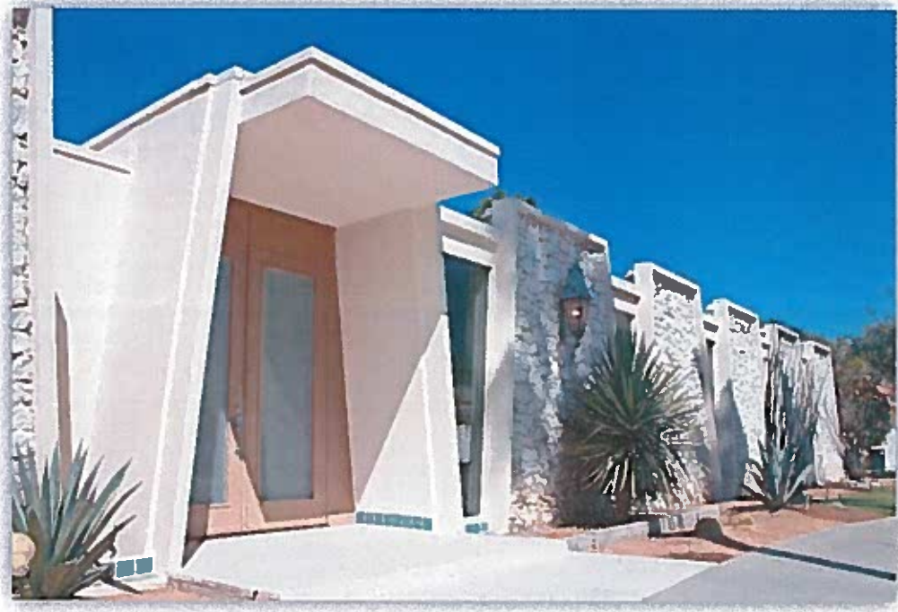
A circa 2005 photograph showing the "unsympathetic" framed glass doors which replaced the original doors. These doors were later replaced in October 2016.
