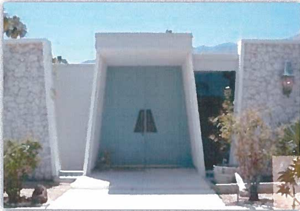
A circa 2004 photograph showing the original solid front doors. Note that the original door pulls were in the shape of an isosceles trapezoid.
