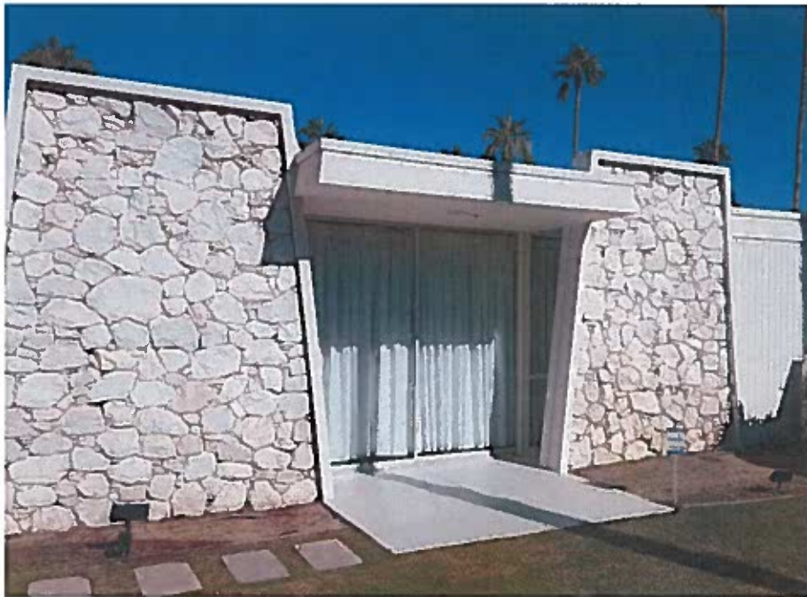
Terrazzo walkway leading to sliding glass doors on south side of residence.
