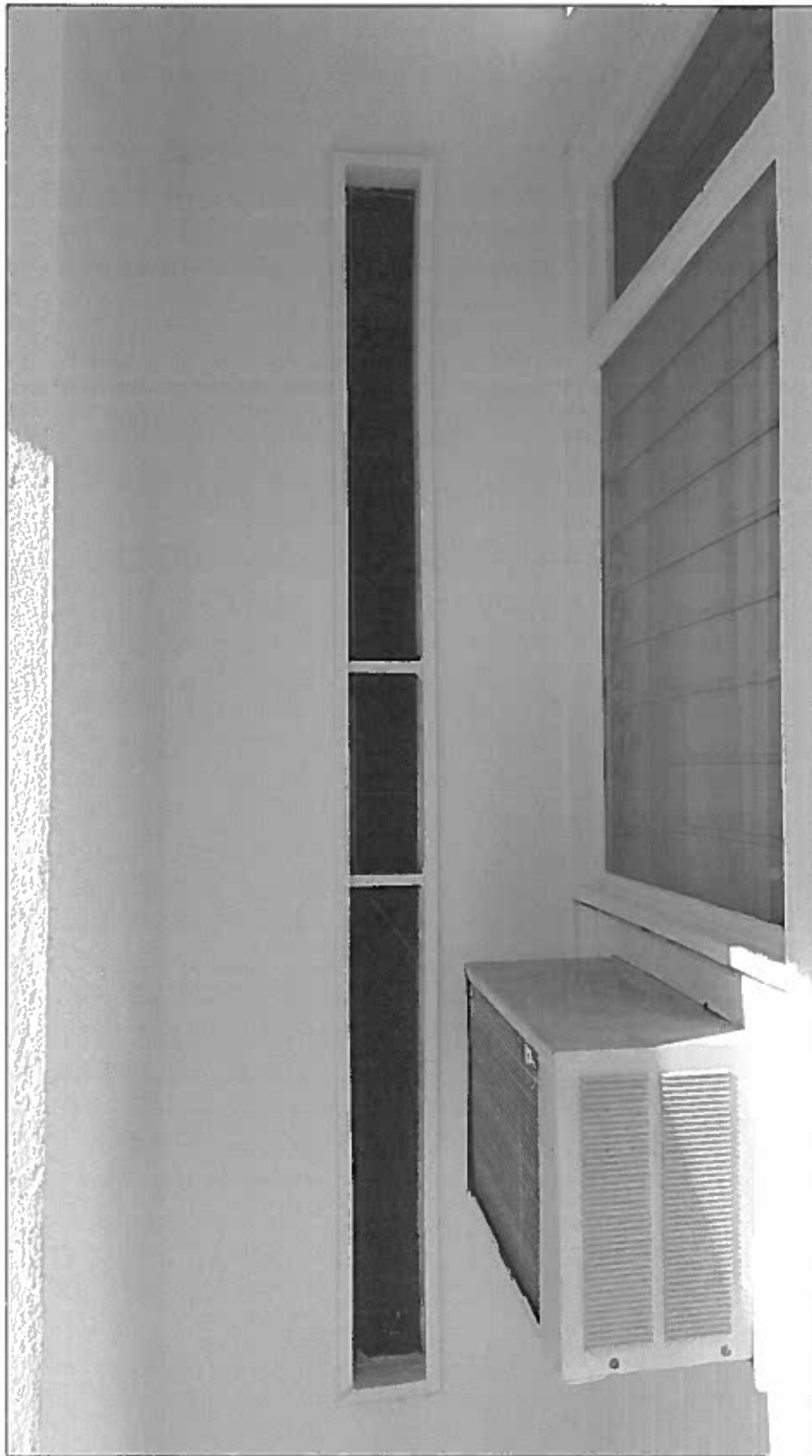
A long vertical window of vintage amber glass is hidden behind a pier on the south side of the residence. Also note that the original jalousie windows were recently covered in glazing (for insurance purposes) in order to retain the feature.
