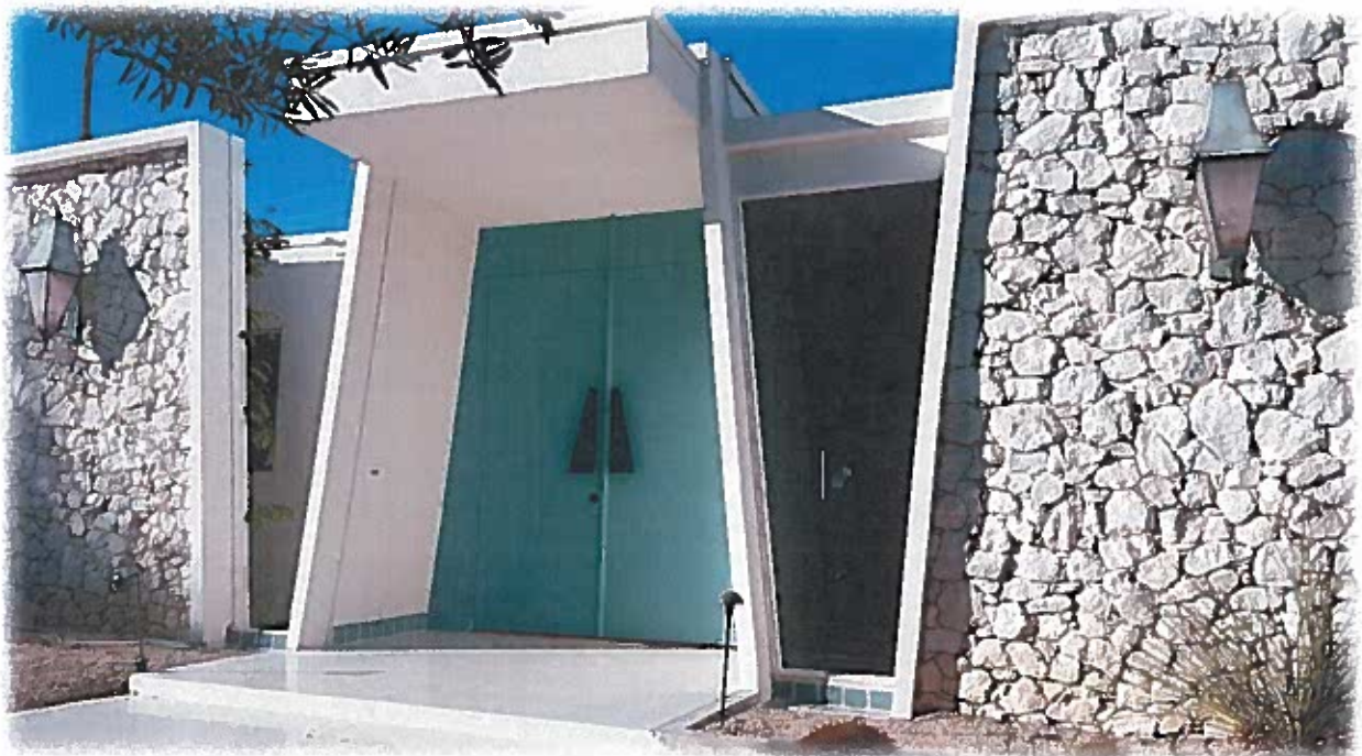
This photograph shows multiple architectural details including (1) a deep, projecting eave over the front doorway, (2) two large copper Hollywood Regency-style lighting fixtures, (3) terrazzo walkway and step, (4) isosceles trapezoidal piers covered in quartzite and (5) glazed turquoise tile at the base of the residence.
