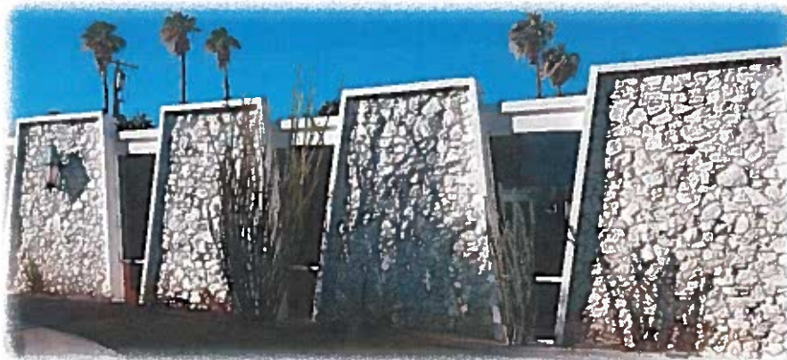
Cofferred stone piers
