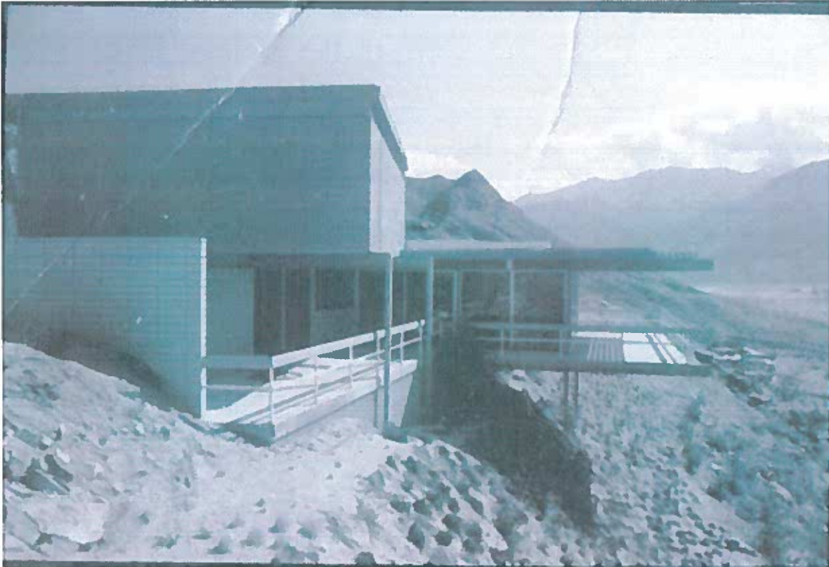
East façade. Original open carport is visible at far left. Hugh Kaptur Collection, Palm Springs Art Museum.
