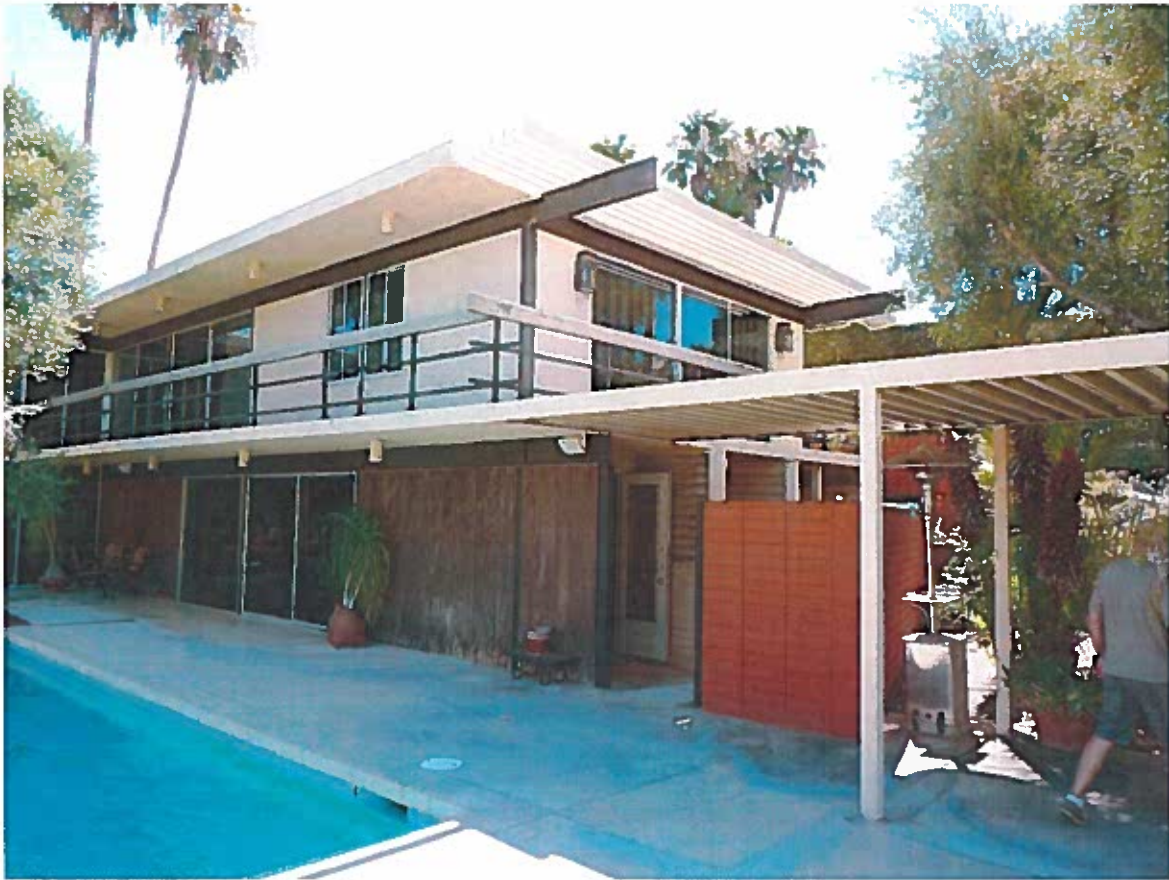
Undated photo of north façade. Steel post-and-beam breezeway to carport addition is also visible at the right of the photograph. Patrick McGrew Collection, Palm Springs Art Museum.
