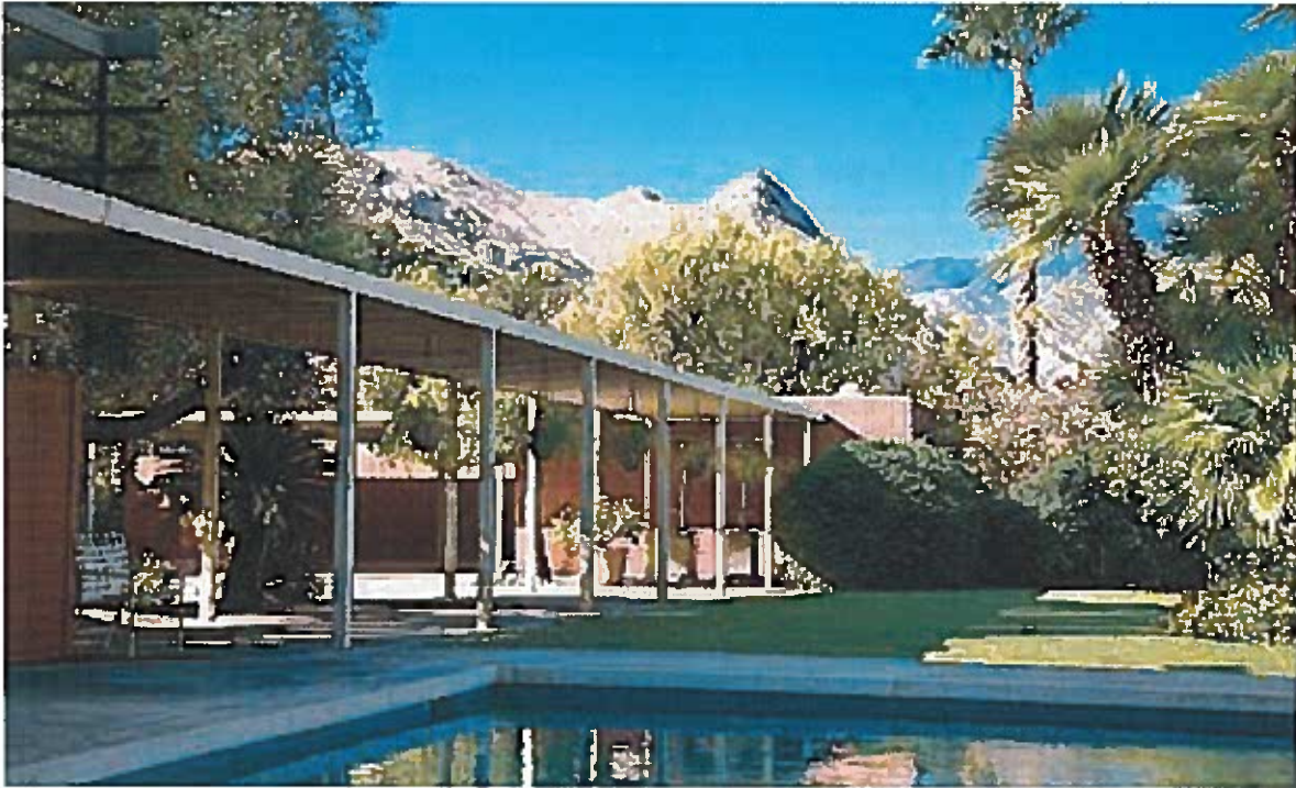
Steel post-and-beam breezeway to new carport addition from 1966. Alison Engel, Palm Springs Life , 2008.
