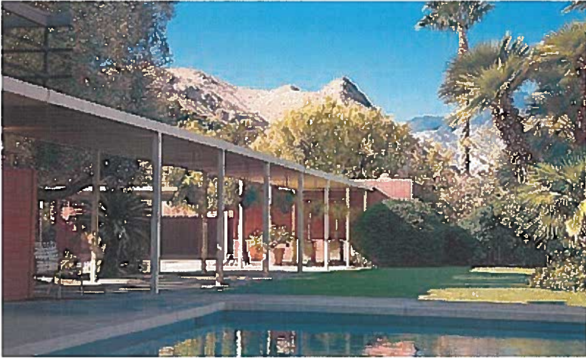
Steel post-and-beam breezeway to new carport addition from 1966. Alison Engel, Palm Springs Life , 2008.
