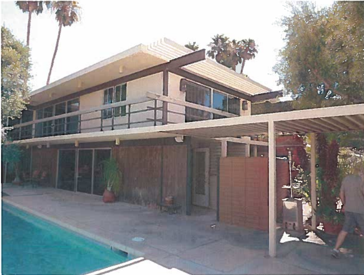
Undated photo of north façade. Steel post-and-beam breezeway to carport addition is also visible at the right of the photograph. Patrick McGrew Collection, Palm Springs Art Museum.
