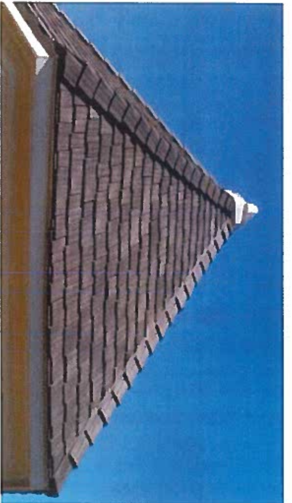
Staggered Enviroshake Roofing
