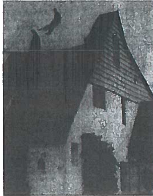
BELOW RT. SHAKE SIDING IN THE GABLE C.1960
