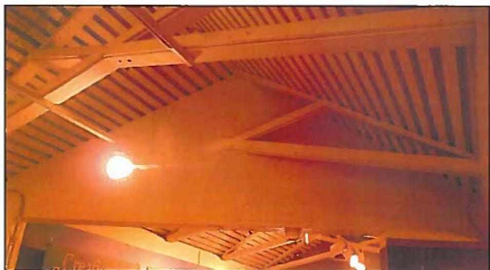
Volume 2 interior, showing detail of scissor truss piercing modern header.
