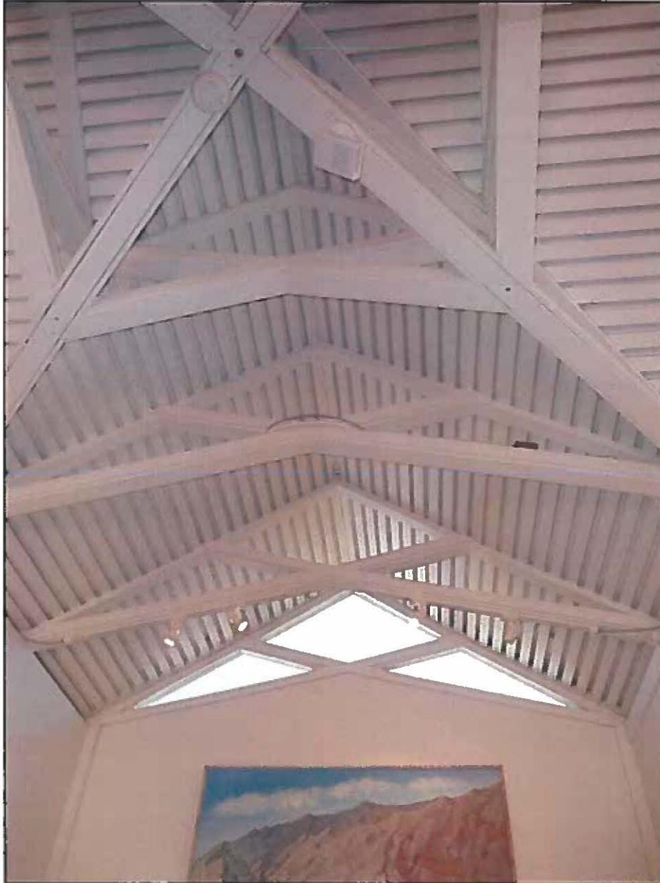
Volume 1 interior, typical scissor trusses and wood slat ceiling.
