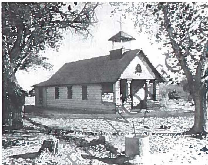
The vernacular St. Florian's Chapel constructed c. 1917 at the corner of East Arenas Road and South Calle El Segundo. Source: Our Lady of Guadalupe website.
