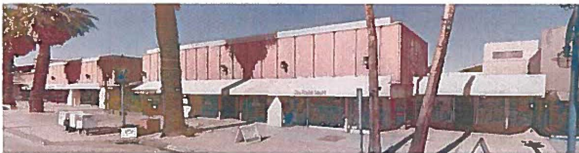
THE MATCHING FACADES OF THE 156-166 BUILDING (FOREGROUND) AND THE 170-174 BUILDING (FAR LEFT)
