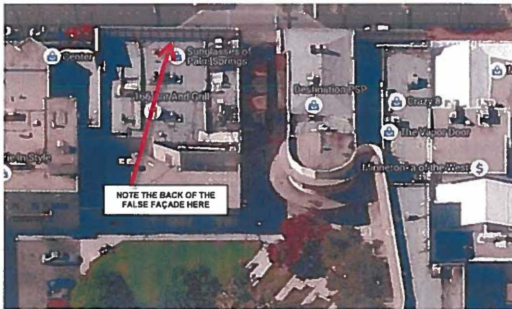
THE AERIAL PHOTO ABOVE SHOWS THE FALSE FAÇADE OF THE 156-166 BUILDING (CENTER LEFT) AND THREE ROOF AREAS OF DIFFERING SLOPES SEPARATED BY LOW PARAPET WALLS. THE 170 BUILDING, WITH THE SEMI-CIRCULAR EAST FAÇADE IS THE ONLY TWO-STORY PORTION OF THE 156 - 174 BUILDINGS.
