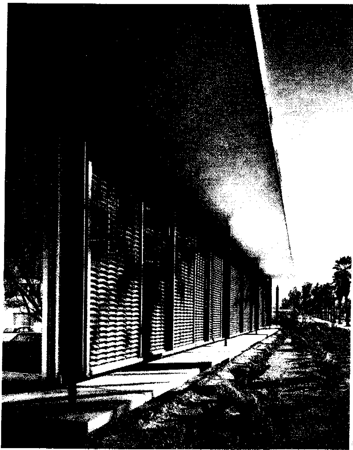
300 South Palm Canyon Drive Santa Fe Federal - West façade, aluminum sunscreens
