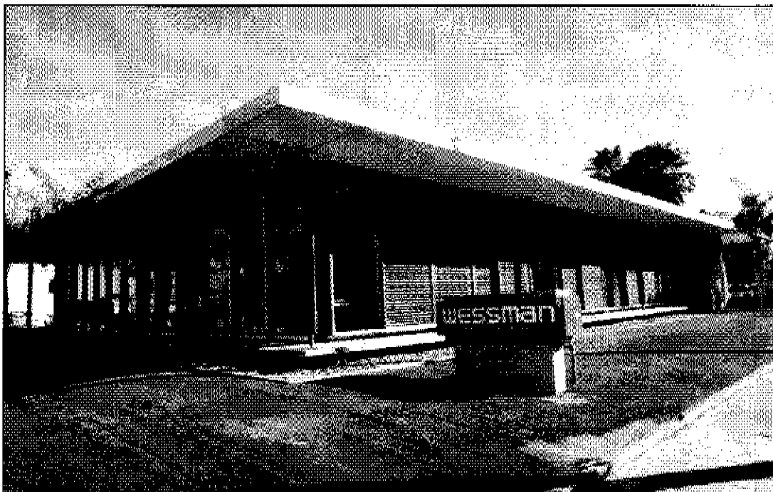
Contemporary Photo of the Santa Fe Federal Savings Bank (Wessman Building)
