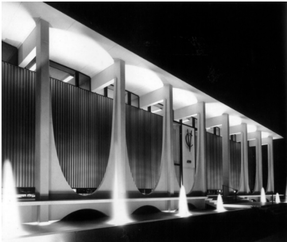
Coachella Valley Savings and Loan #2 (1961, Williams, Williams & Williams). Photographed by Julius Shulman. Source: The J. Paul Getty Research Institute, Los Angeles. Digital Photo Collection.
