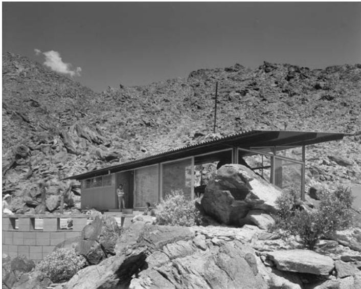
Frey House II (1963, Albert Frey; HSPB-33, listed in the National Register). Photograph by Julius Shulman. Source: The J. Paul Getty Research Institute, Los Angeles. Digital Photo Collection.
