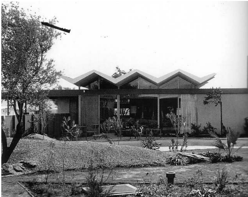
Rear façade of the steel house with folded plate roofline (1961-62, Donald Wexler or Wexler & Harrison). Source: Steel and Shadow: The Architecture of Donald Wexler , 23.
