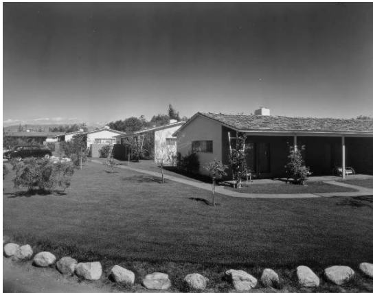
Racquet Club bungalows designed by Clark & Frey in 1948. Photographed by Julius Shulman. Source: The J. Paul Getty Research Institute, Los Angeles. Digital Photo Collection.
