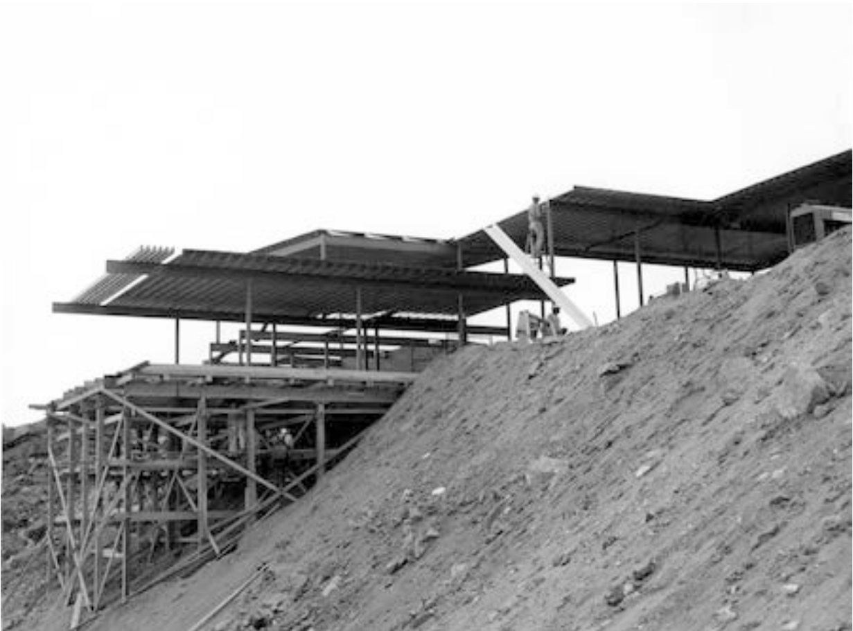
The post-and-beam Morris House (1964, Hugh Kaptur) under construction on a hillside site in Southridge Estates. Source: Palm Springs Life Archives .
