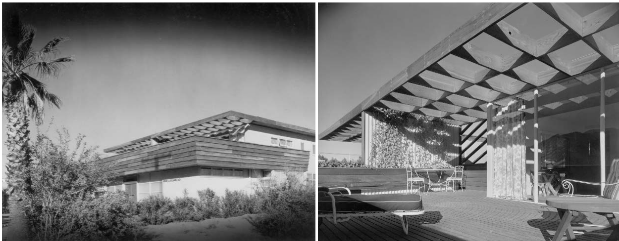
L: Potter Clinic (1947, Williams, Williams & Williams; HSPB-58) located at 1020 N. Palm Canyon Drive. The combination retail and residential apartment building was, according to Julius Shulman, where architect E. Stewart Williams lived in 1949. R: The apartment featured a dining patio that was accessible from the kitchen. The redwood trellis protected the glassed in dining area from the late afternoon sun in the southwest. Photographs: Julius Shulman. Source: The J. Paul Getty Research Institute, Los Angeles. Digital Photo Collection.
