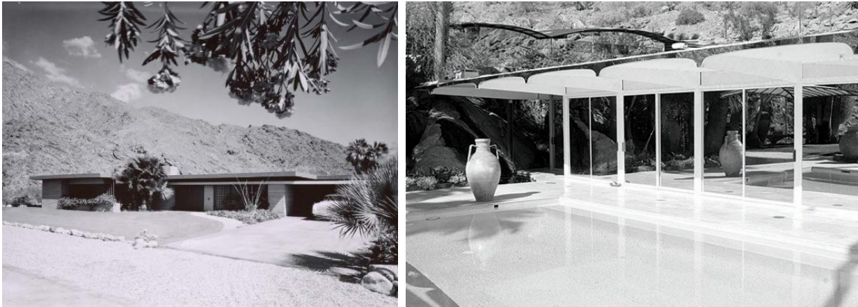
L: Crockett House (1956, Herbert Burns). Photograph by Julius Shulman. Source: The J. Paul Getty Research Institute, Los Angeles. Digital Photo Collection. R: Burgess House (1958, Hugh Kaptur). Source: Palm Springs Life , "Ready for their Close-ups." Photographer Jay Jorgensen.
