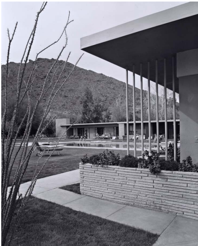
L: The one-story Town & Desert Apartments (c.1948, H.W. Burns; HSPB-90) at 370 W. Arenas Road features an L-shaped Mid-century Modern design oriented toward the swimming pool. Photograph: Julius Shulman. Source: The J. Paul Getty Research Institute, Los Angeles. Digital Photo Collection. R: Ad for Town & Desert Apartments indicates the designer and his wife were also managing owners of the project. The architecture and the location were the clear stars of this ad. Source: Villager , November 1952, 8.
