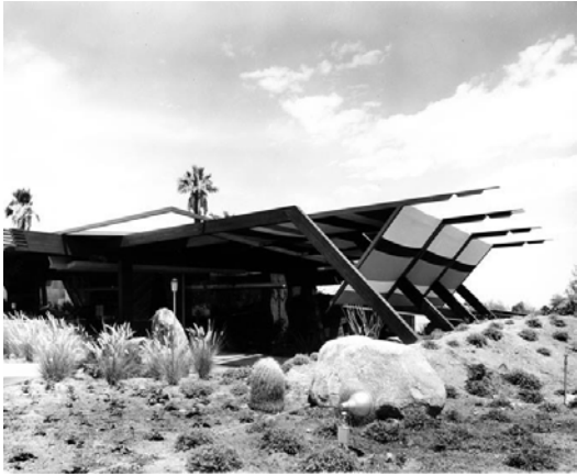
The Huddle Springs restaurant (1956, William Cody; demolished). Source: Lost Palm Springs.
