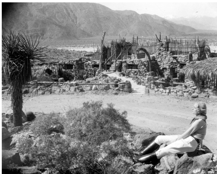
Little Araby Rock House. Source: Los Angeles Public Library.
