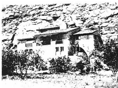
One of the Homes We Have Built
