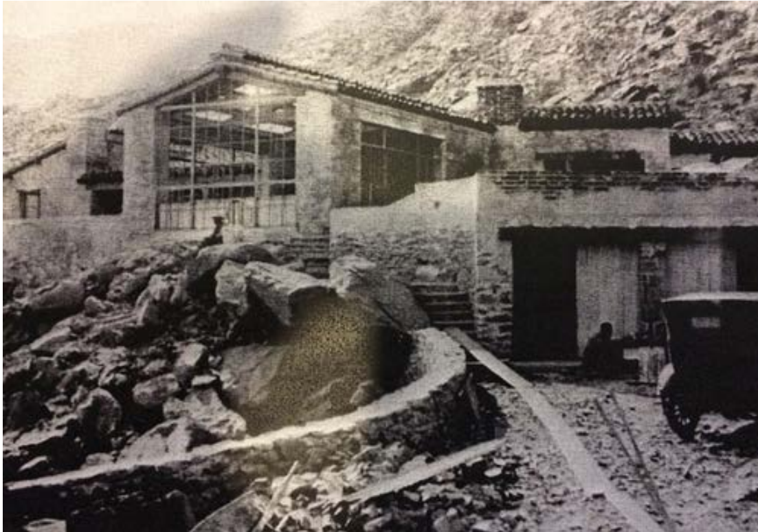
Burnham House, completed in 1929. Part of a group of buildings on S. Tahquitz Drive that comprised an artists' colony. Source: Colony 29 website.
