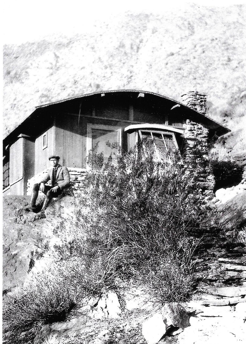
Avery Edwin Field sits in front of his cabin, ca. 1922. Note the interesting architectural details including the atelier window, barrel roof, stacked-stone chimney and stone steps leading up from the Tahquitz Ditch.
