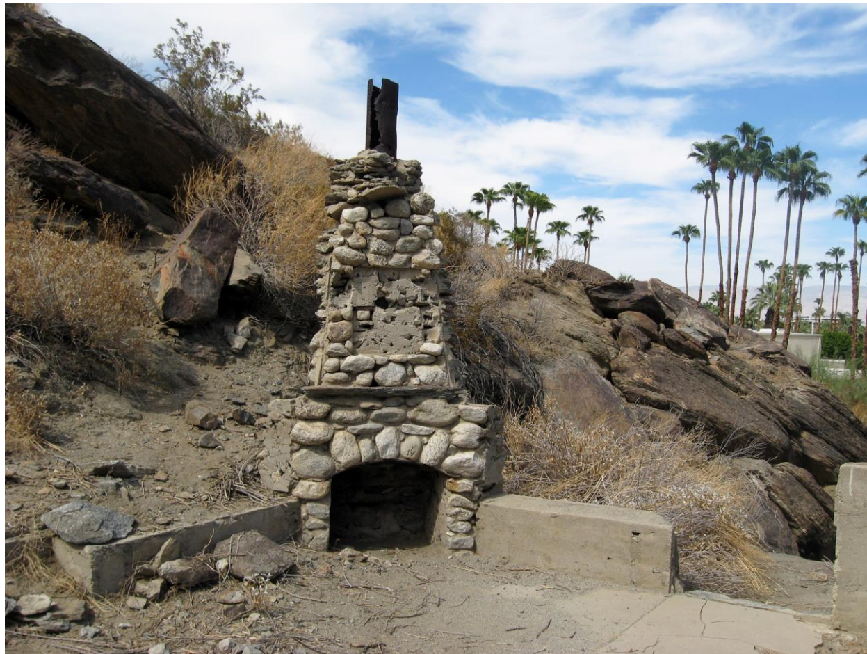
Field Cabin fireplace. Note indented section where a plaque or painting may have been held and mantel of desert varnished granite. Tennis Club is in the background. (Author photo. August 2018)
